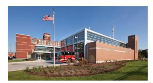
This new 20,063-square-foot Engine Company 16 firehouse features load bearing masonry with exterior brick finish and has been designed to last 100 years, constructed of durable materials that will stand the test of time and the impact of being a 24-hour facility. The facility also includes:
