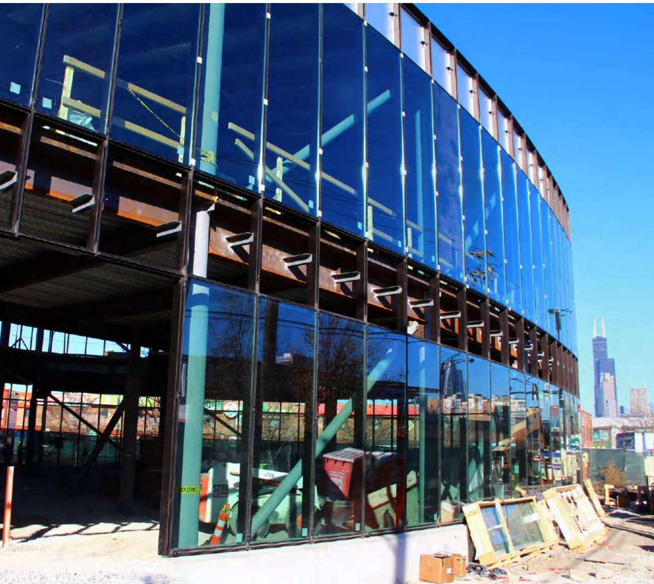
Construction at the Chinatown Branch Library.
