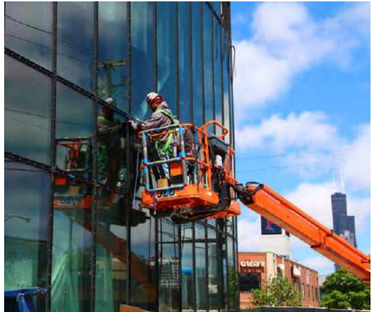
A worker installs windows at Chinatown Branch Library.
