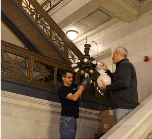
As part of Retrofit One, workers at the Cultural Center upgrade light fixtures with energy-efficient bulbs.
