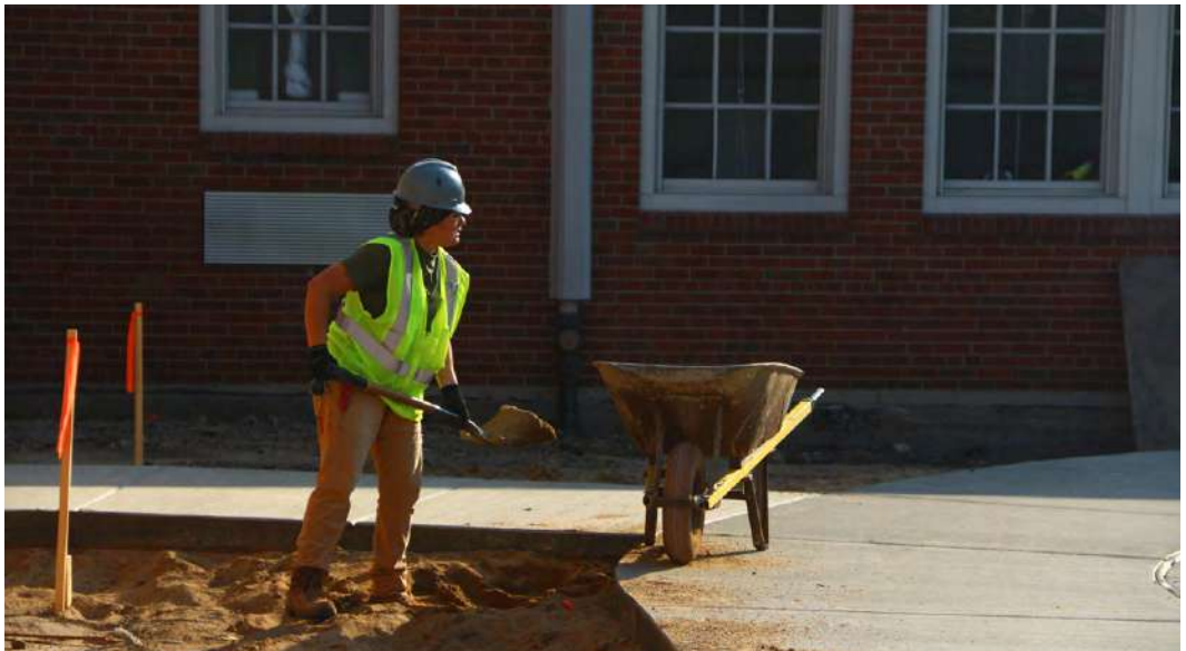
Work is underway at Wildwood World Magnet School Annex.
