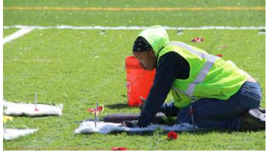
A community resident installs yard numbers on the turf field at National Teachers Academy.
