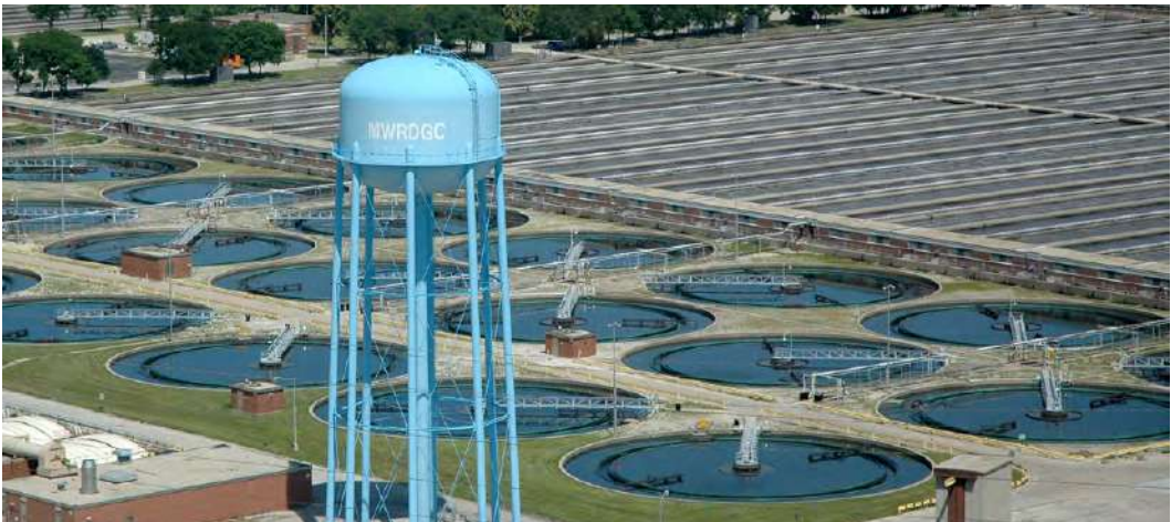
The MWRD's Stickney Wastewater Treatment Center.
