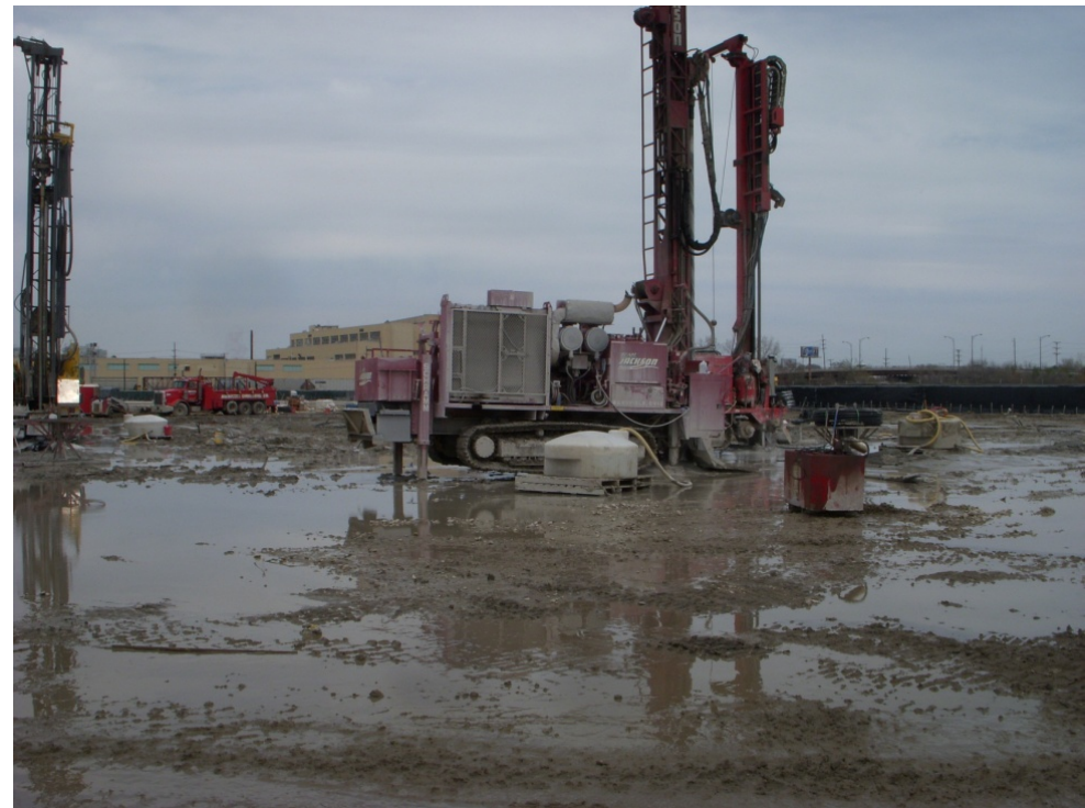
Drilling wells for geo-exchange system
