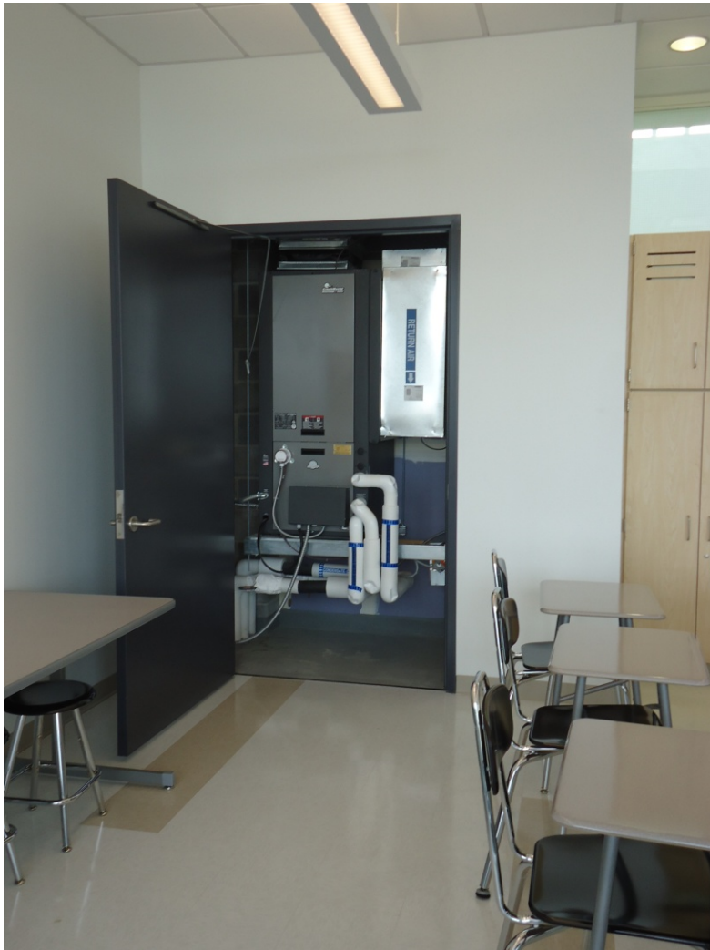
Heatpump Closet located in classroom
