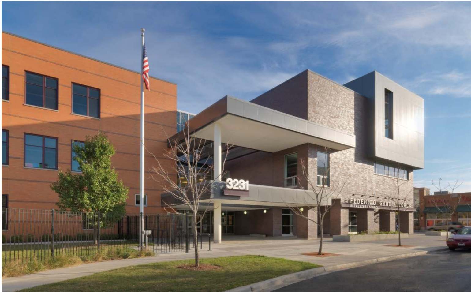
Federico Garcia Lorca Elementary School
