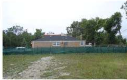
VIEW SOUTHEAST - RESIDENTIAL
