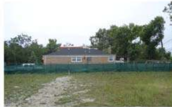
VIEW SOUTHEAST - RESIDENTIAL
