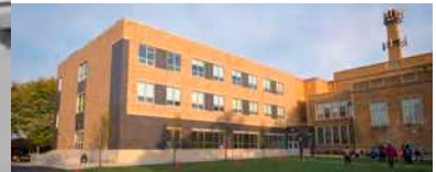
Jamieson Elementary School Annex LEED Silver
