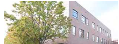
Edwards Elementary School Annex LEED Silver
