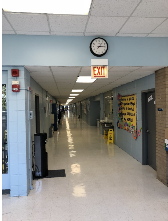
Photo 30 View of main corridor looking south. Interior partitions walls are typically CMU typically with dropped hard ceiling soffits at the classroom entries. See also Roof Assessment Report as corridor ceiling shows significant signs of leaking.
