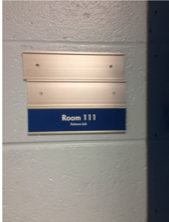
Photo 38 View of classroom signage. Interior signage is not ADA compliant.
