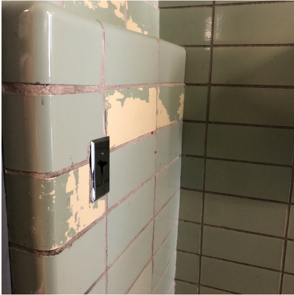
Photo 35 Spalled and deteriorated pointing at the glazed CMU at the student toilet rooms.
