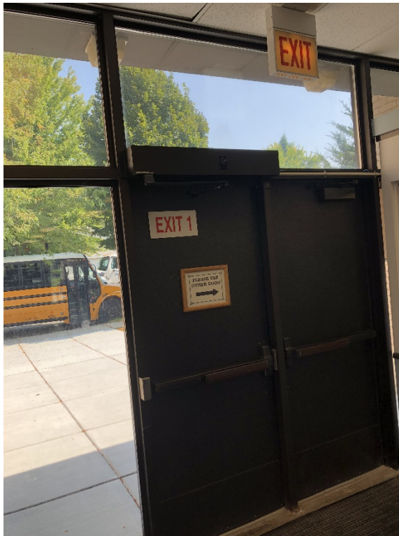
Photo 21 View of main entry looking east. Entry includes an ADA automatic door operator and AI Phone equipment.
