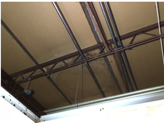
Photo 41 View of roof joists above corridor ceiling. Roof leaks were visible at numerous locations along the corridor.
