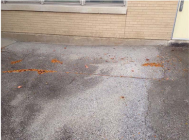
Photo 8 Apparent UST excavation.
