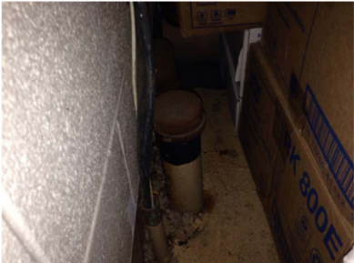
Photo 7 Apparent UST piping.
