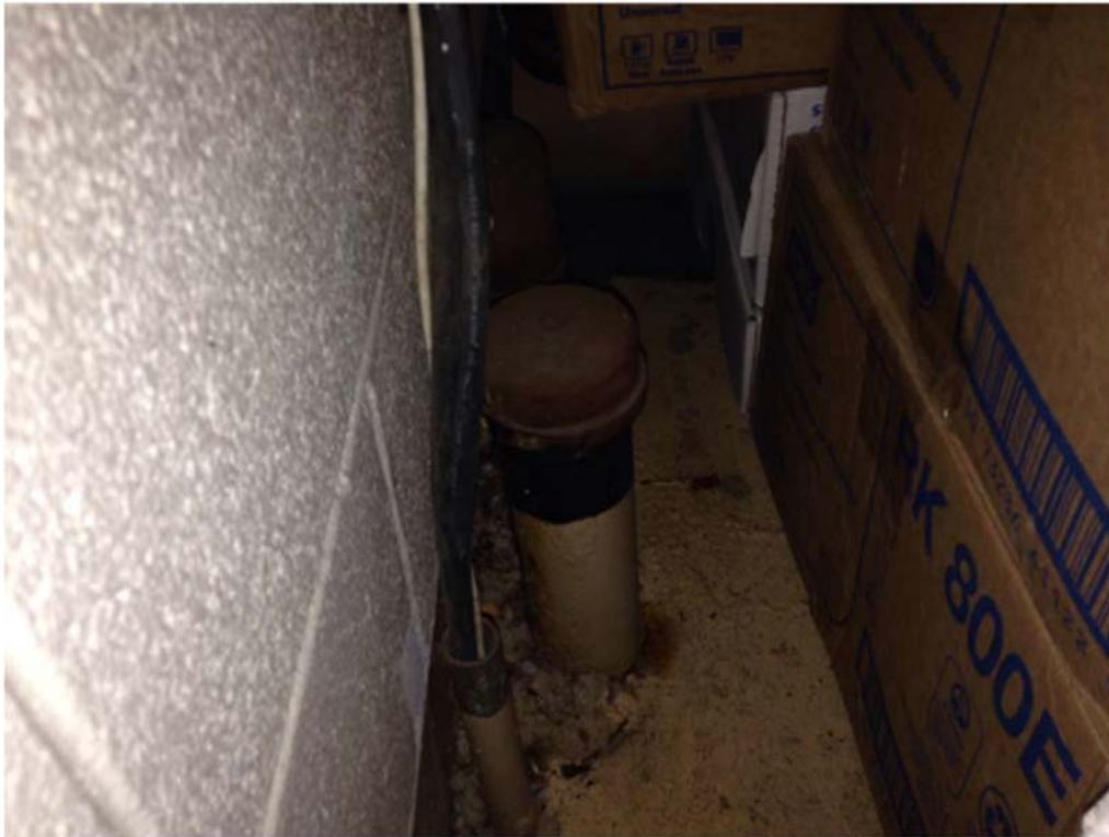
Photo 7 Apparent UST piping.
