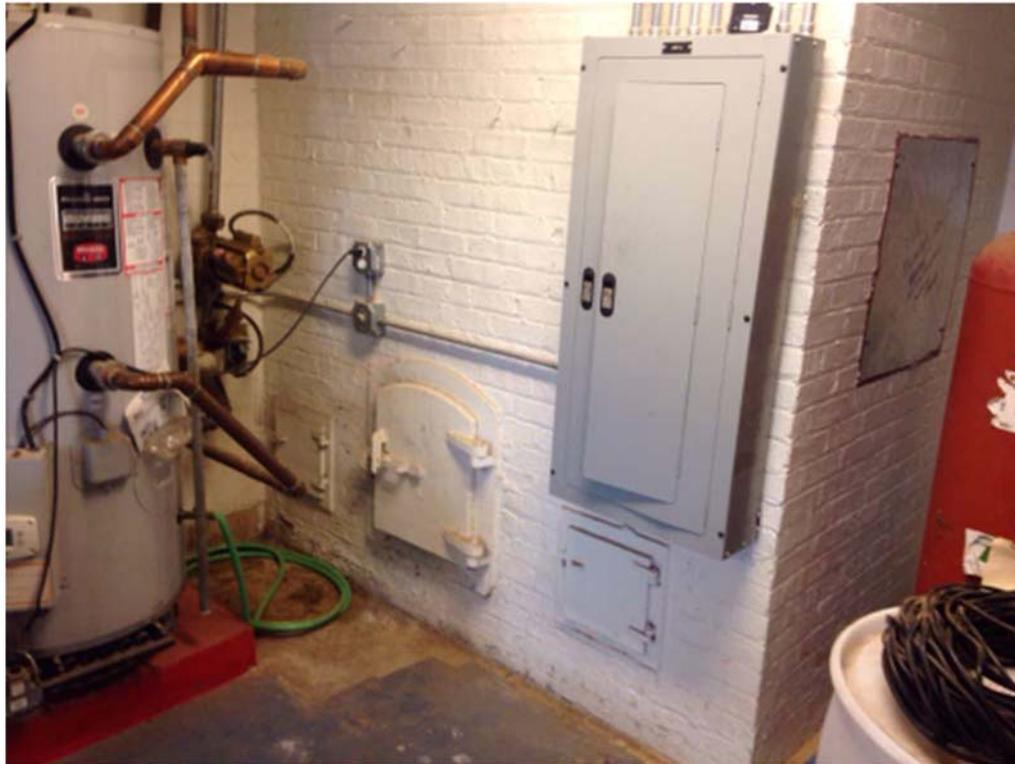
Photo 1 Incinerator in mechanical room.
