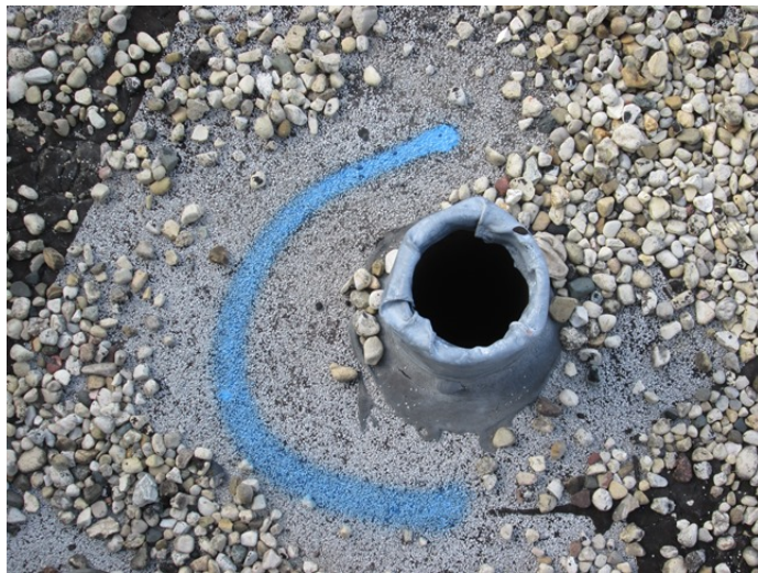
18. CLOGGED SOIL STACK
