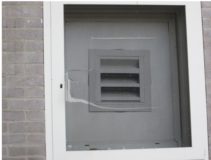
20. DAMAGED SCREEN
