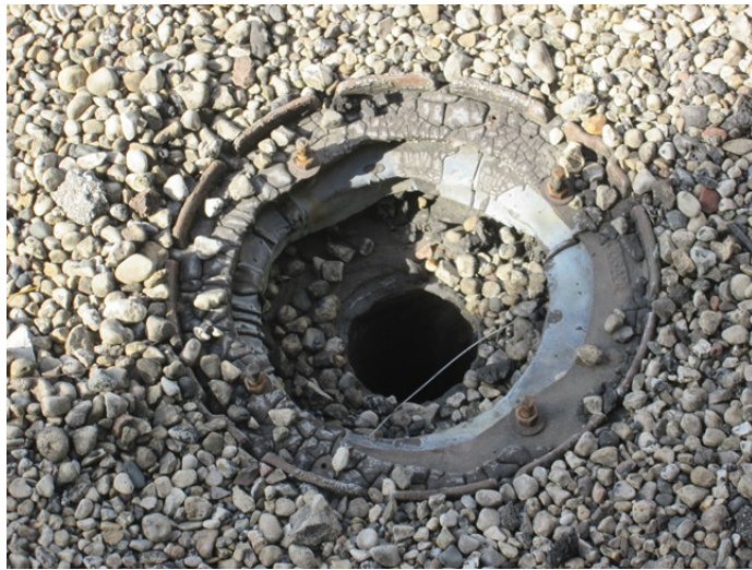
17. MISSING DRAIN STRAINER
