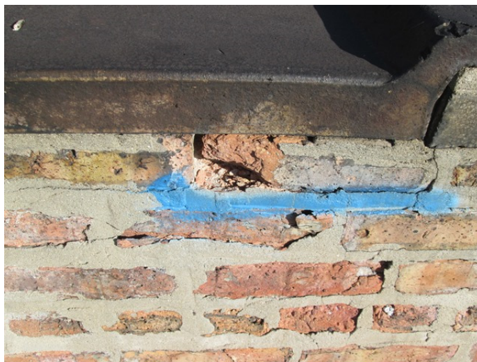
12. DETERIORATED MASONRY
