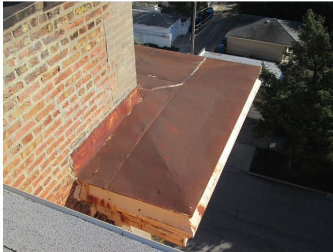
13. DETERIORATED CORNICE (TYPICAL)
