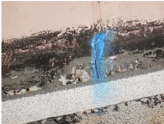
5. DAMAGED METAL FLASHING
