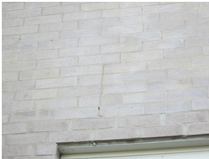
23. CRACKED MASONRY
