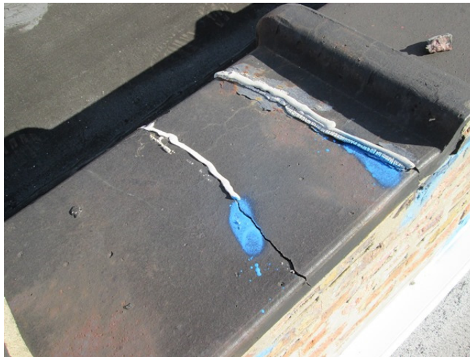
14. DAMAGED COPING TILES
