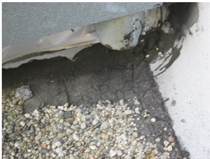
21. MISSING SPLASH BLOCK
