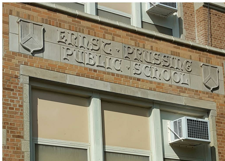
EXAMPLE OF CNC LIMESTONE LETTERING - REPLACEMENT FOR CRUMBLING TERRA COTTA
