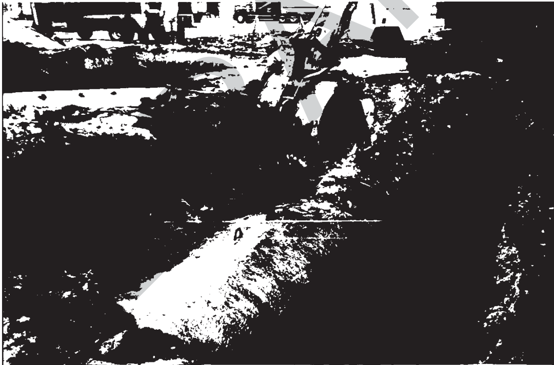
PHOTOGRAPH 4: UST No. 9 being opened up for cleaning, UST No. 2 at left.
