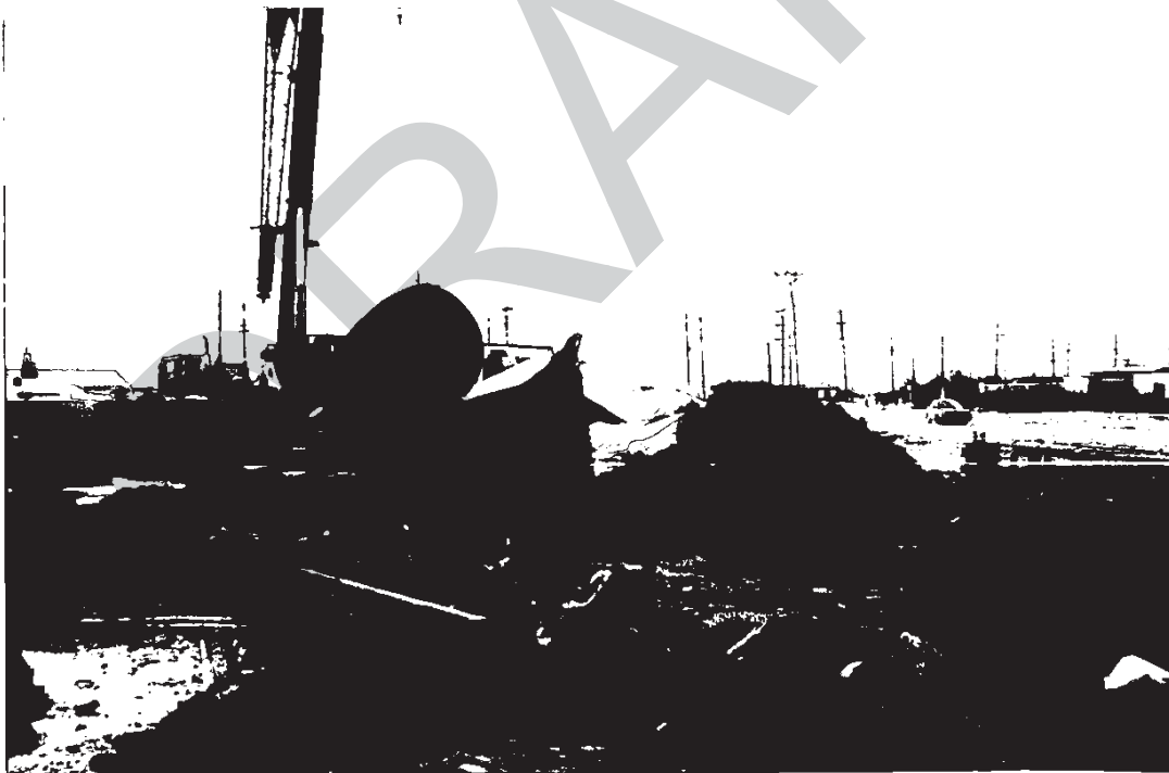
PHOTOGRAPH 6: UST No. 9 being pulled out of excavation by crane.
