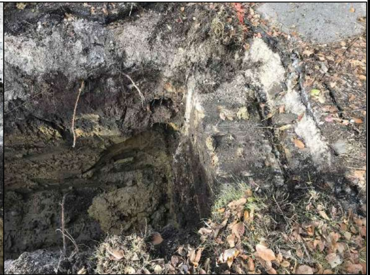
38: TP-30, wall footing, view west
