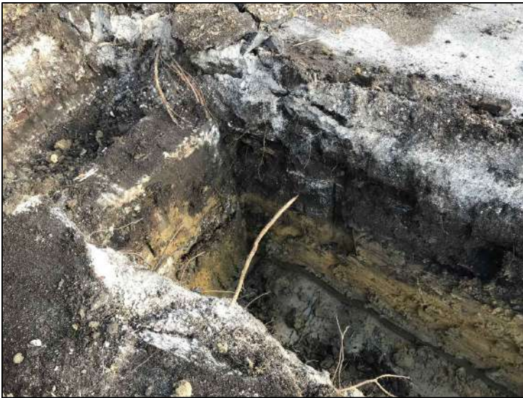
37: TP-29, wall footing, view east
