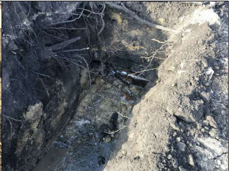
16: TP-13, probable abandoned water main, view north
