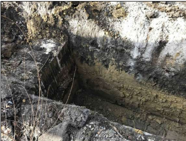
39: TP-31, wall footing, view east
