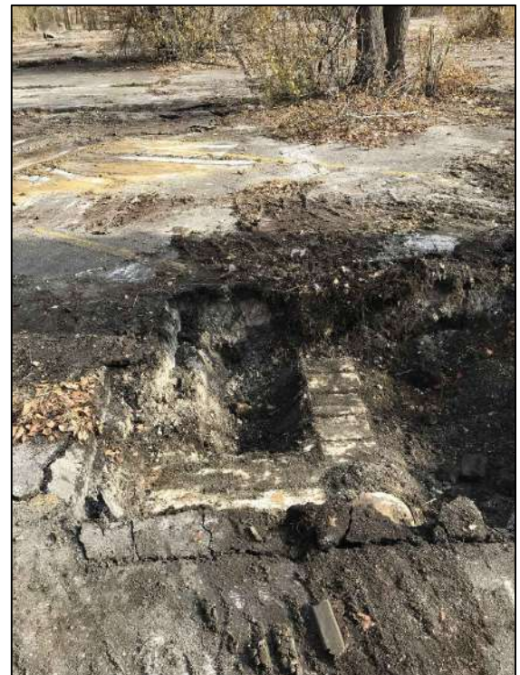
28: TP-22B, corner wall footing, view east
