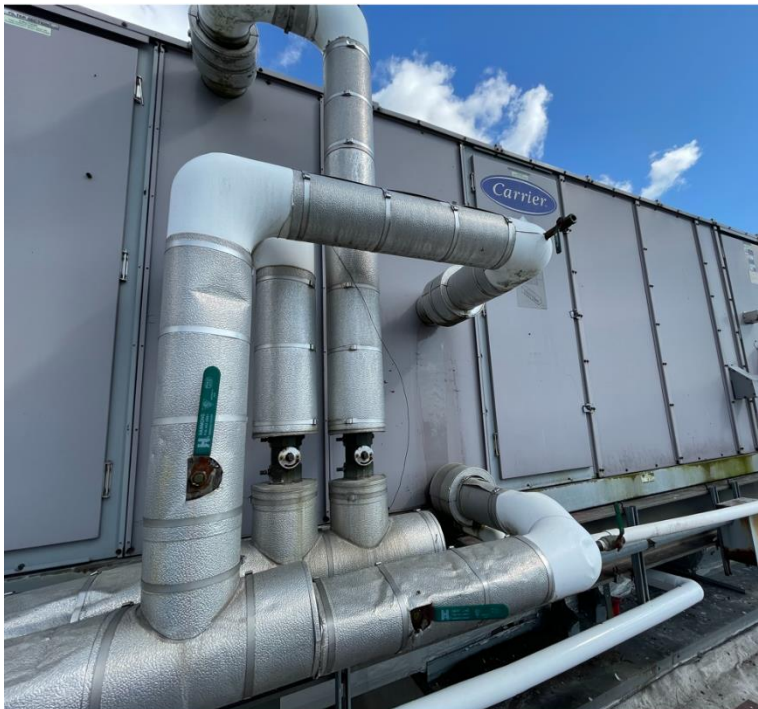
Existing RTU-1 Cooling coil leaking
