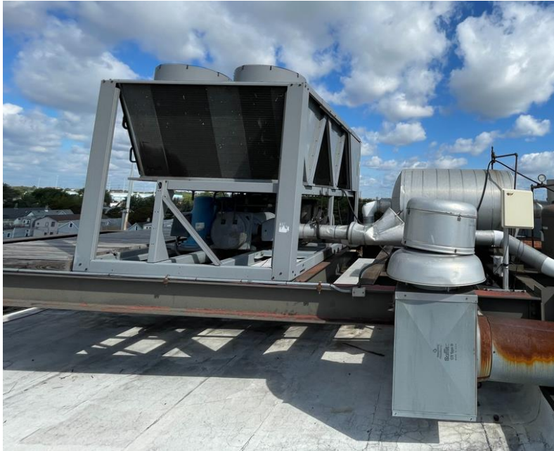
Existing Air-cooled chiller system CH-1
