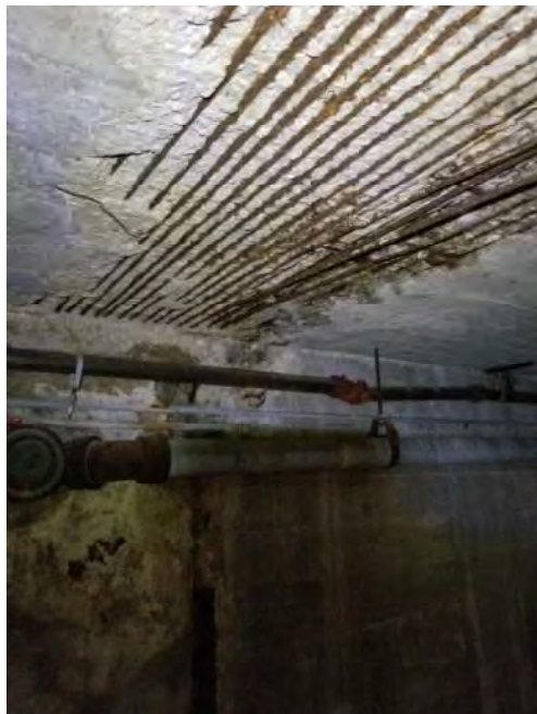
Exposed Rebar in Tunnel Roof Slab
