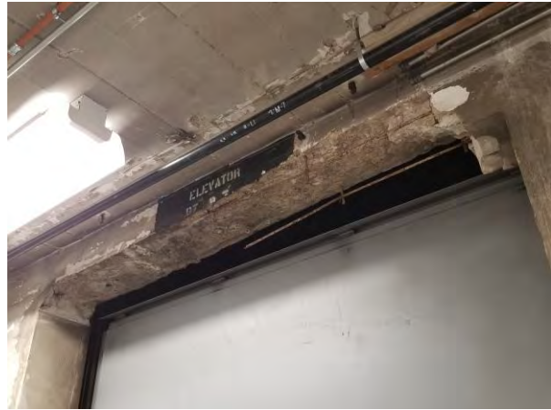
Cut Beam at Elevator B6
