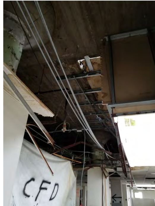
Water Damage at Skylights
