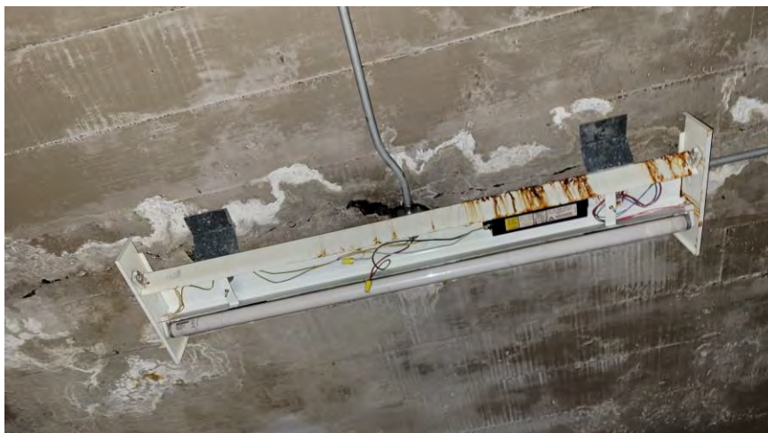
Cracking @ Water Infiltration in Floor Slab
