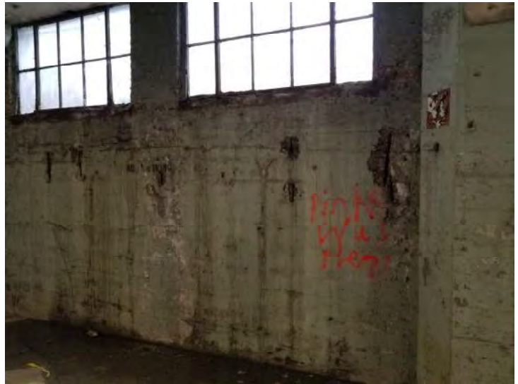
Exposed Rebar in Basement Wall
