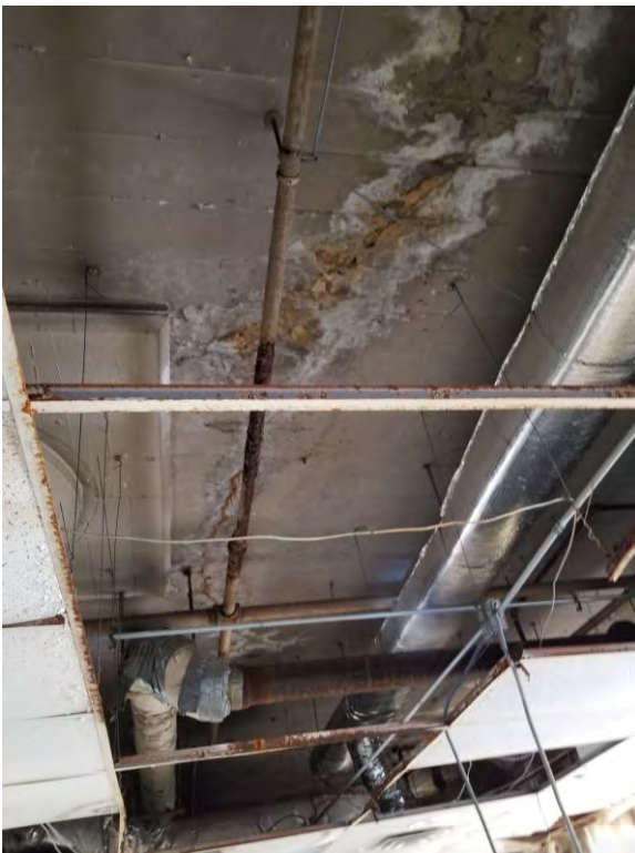
Corrosion visible on underside of Roof slab
