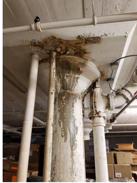
Water Damage at Column
