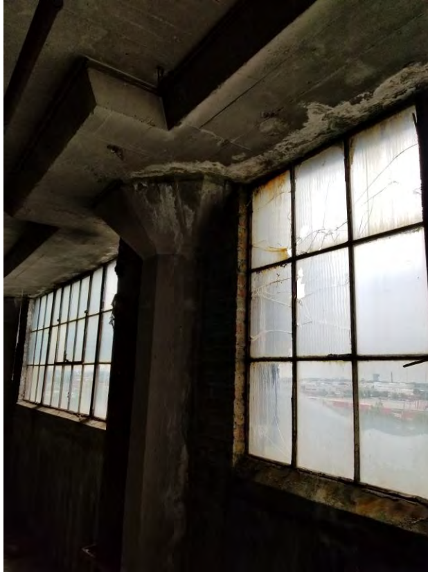
Deterioration of spandrel beam on north side of building
