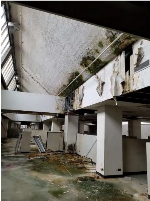
Water Damage at Skylights
