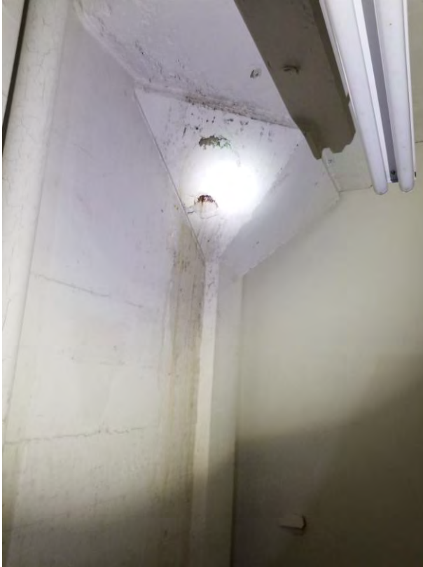
Active leak through column capital
