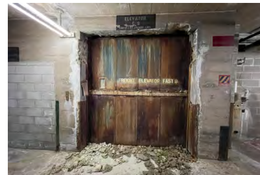
E - Elevator Lintel Deterioration
