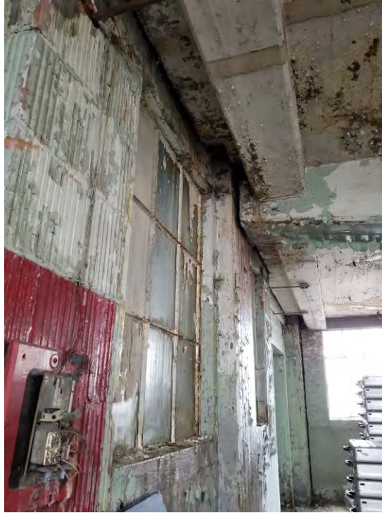
Water Damage at Expansion Joint between Main Building and Interconnecting Bridge
