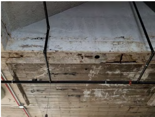
Exposed Rebar around Skylight
