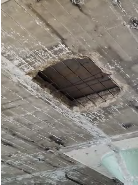
Cut Slab Near Column M.2
