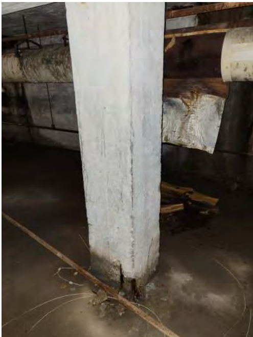
Concrete Post in Tunnel with Exposed Rebar
