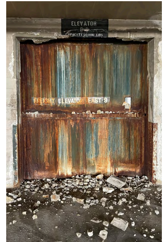
C - Deteriorated Lintel Elevator 9
