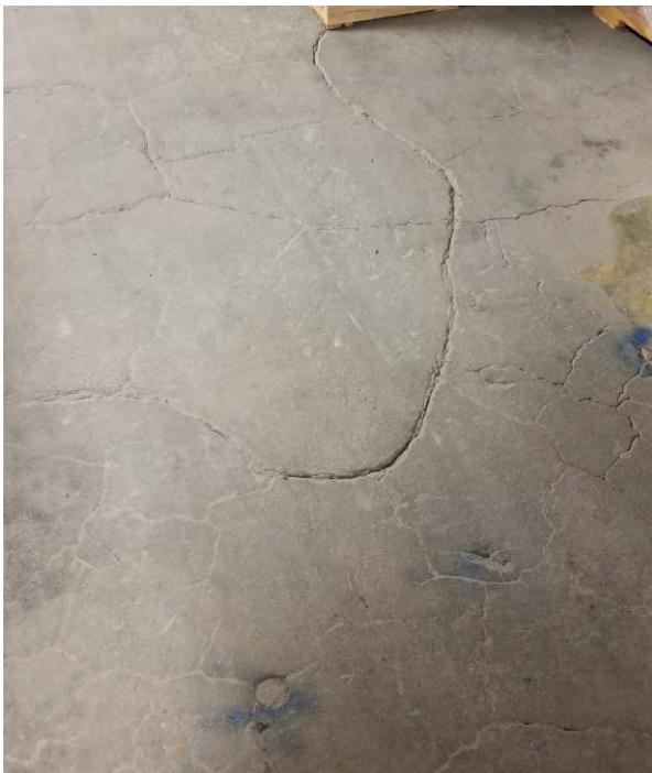
Floor Cracks at Level 5
