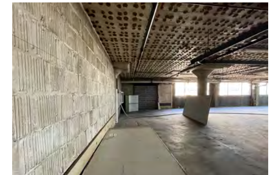
D - Masonry fill at existing bridge
