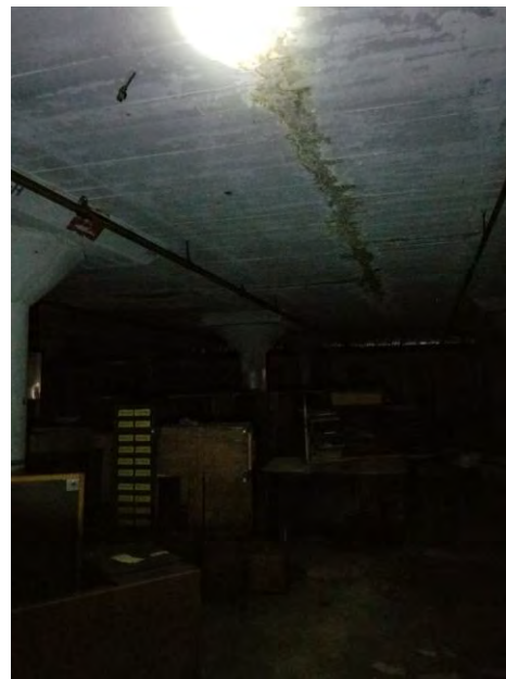
Continuous Crack at Slab Underside
