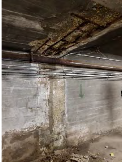
Deterioration in Underside of Link Slab
