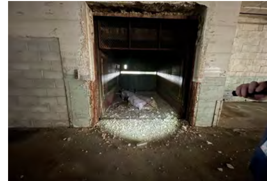
B - Deteriorated Lintel Elevator 9
