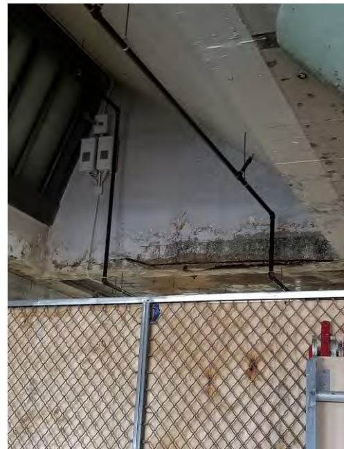
Exposed Rebar around Skylight
