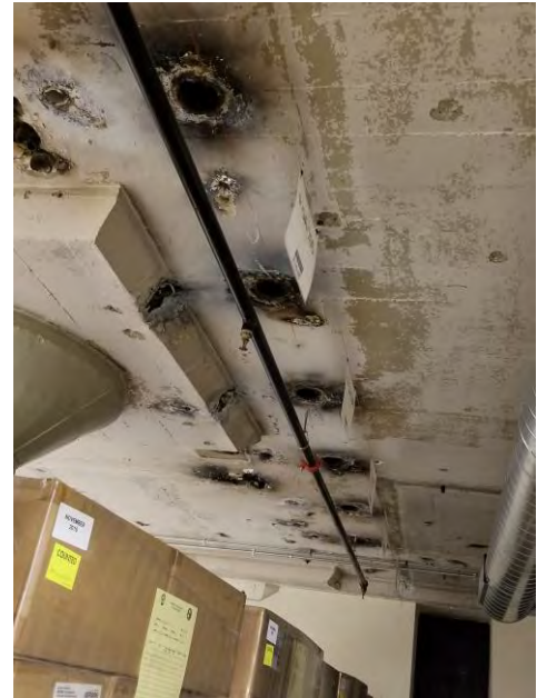
Plumbing Cores Through Concrete Slab
