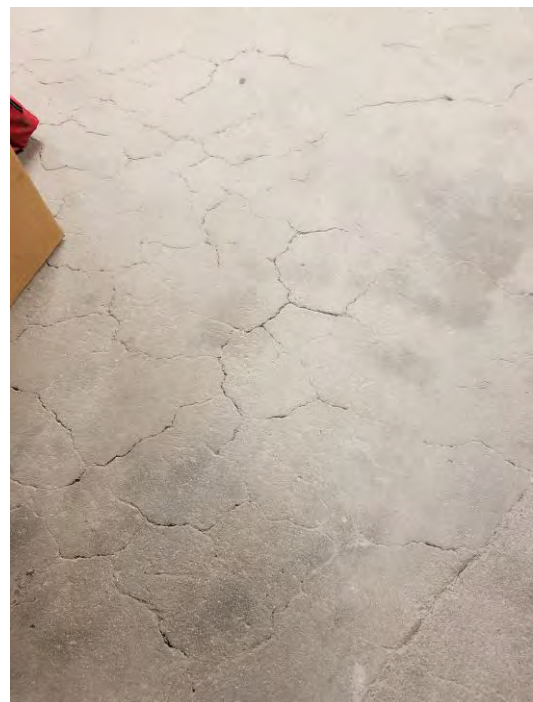
Floor Cracks at Level 5
