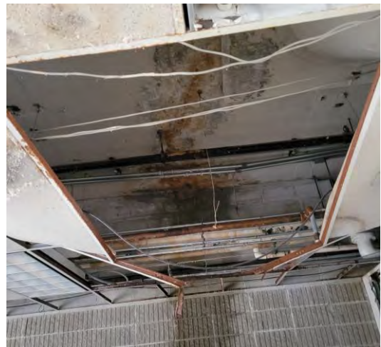
Water Damage and Cracking in Roof Slab
