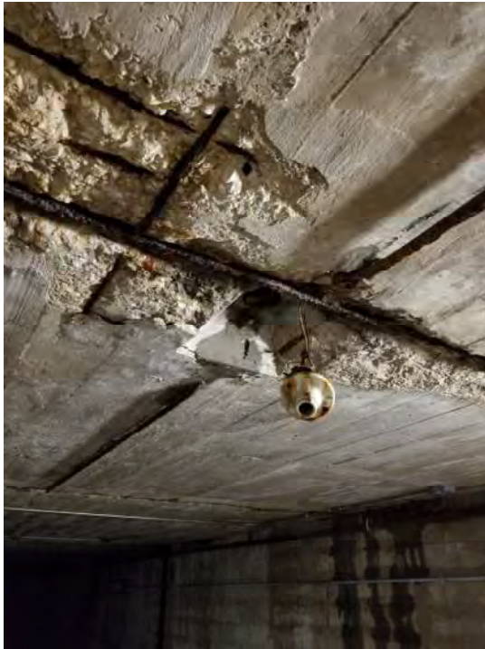
Exposed Rebar in Tunnel Slab
