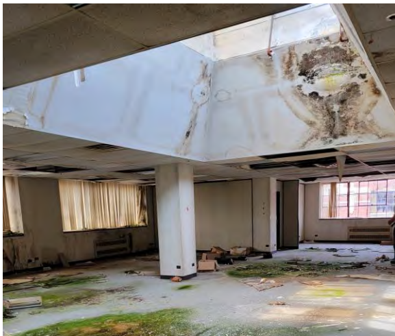
Mold and Corrosion @ Skylight
