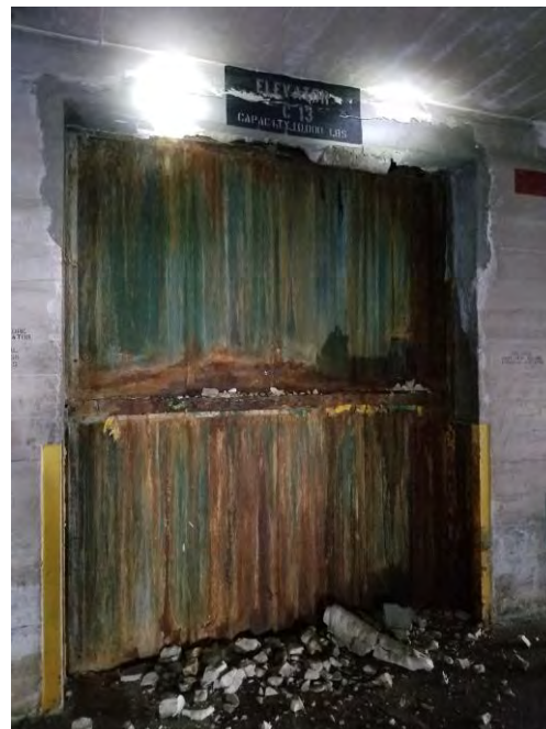
Elevator 13 Spalled Concrete
