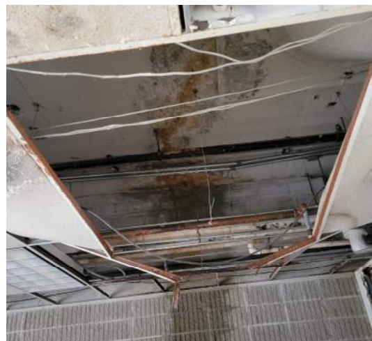
Water Damage and Cracking in Roof Slab
