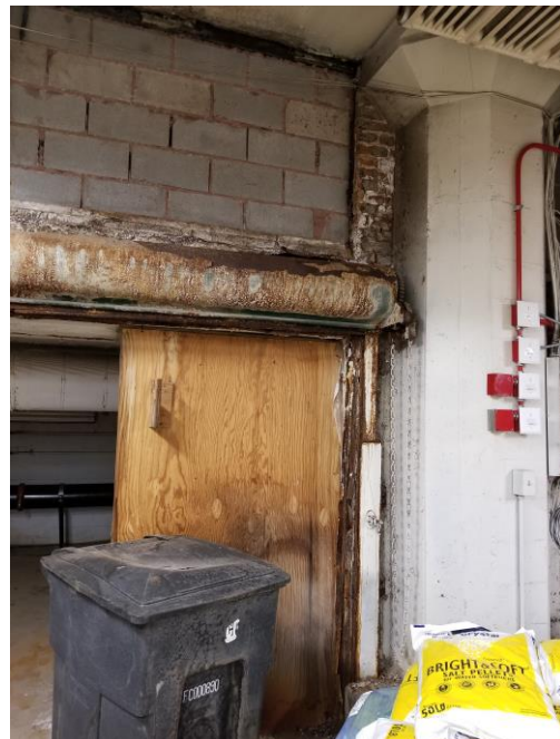
Deteriorated Masonry at Tunnel Entrance
