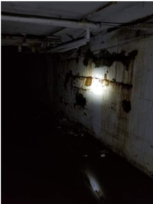
Deteriorated Rebar in West Building Tunnel
