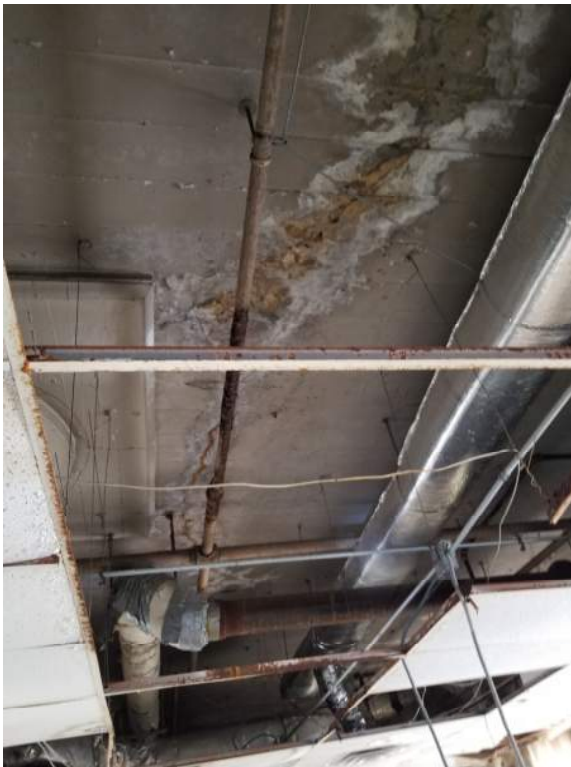
Corrosion visible on underside of Roof slab
