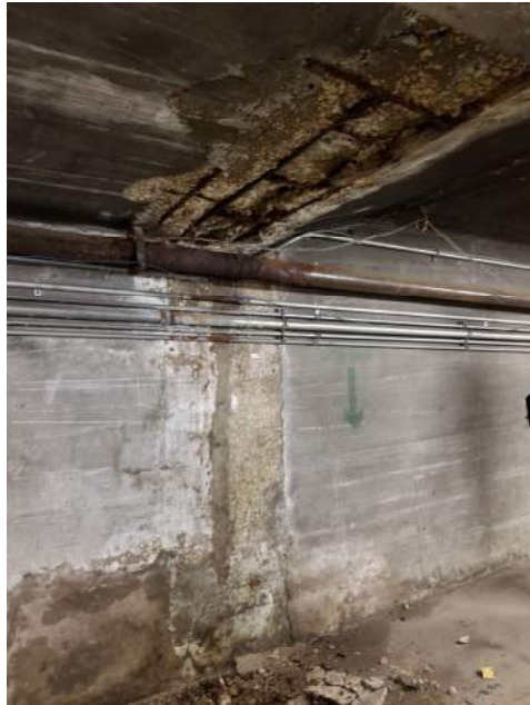
Deterioration in Underside of Link Slab
