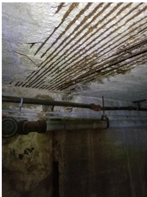
Exposed Rebar in Tunnel Roof Slab
