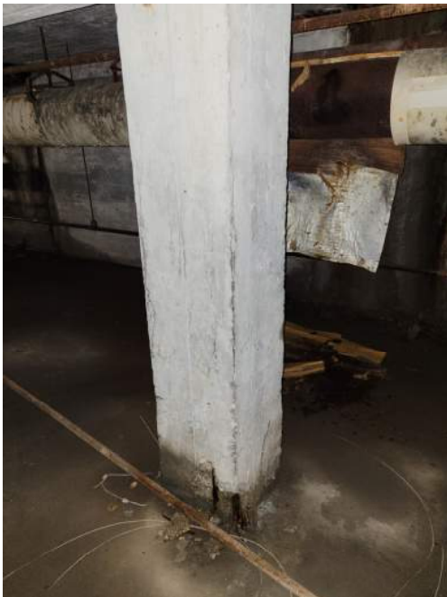
Concrete Post in Tunnel with Exposed Rebar
