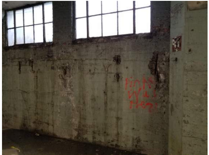
Exposed Rebar in Basement Wall
