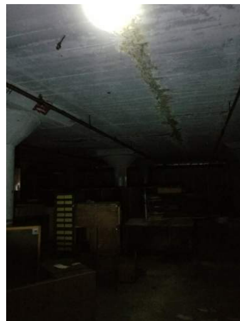
Continuous Crack at Slab Underside
