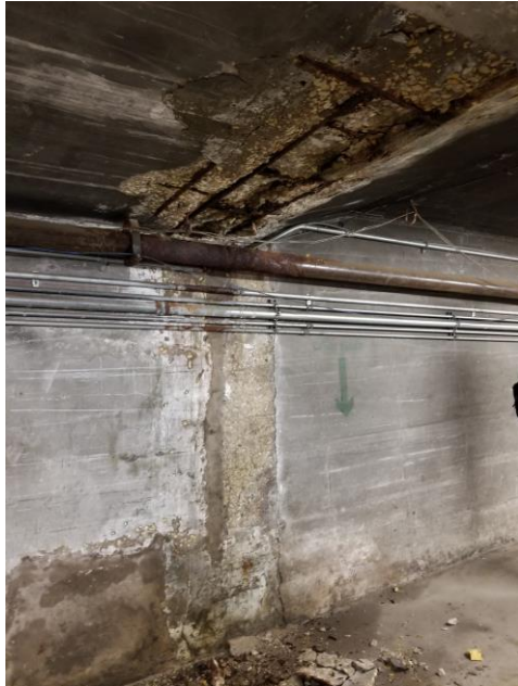
Deterioration in Underside of Link Slab
