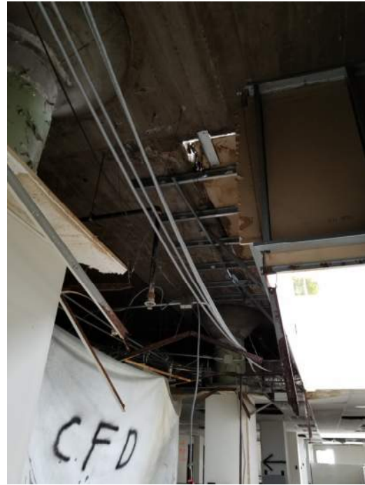
Water Damage at Skylights
