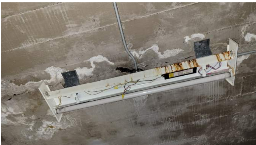
Cracking @ Water Infiltration in Floor Slab
