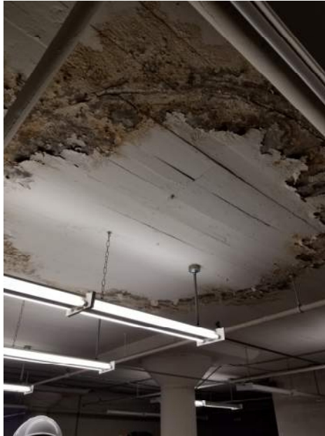
Level 5 Water Damage
