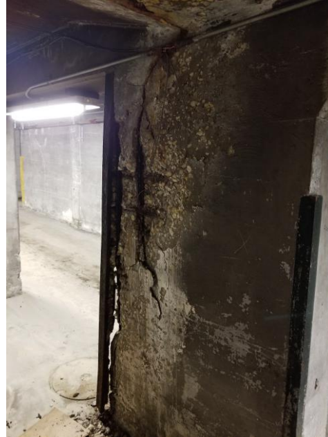
Deterioration of Link Column
