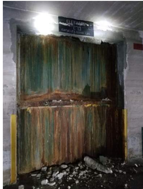
Elevator 13 Spalled Concrete
