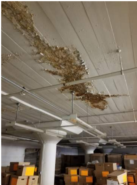
Level 5 Water Damage
