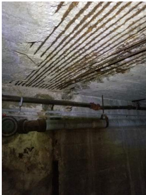
Exposed Rebar in Tunnel Roof Slab
