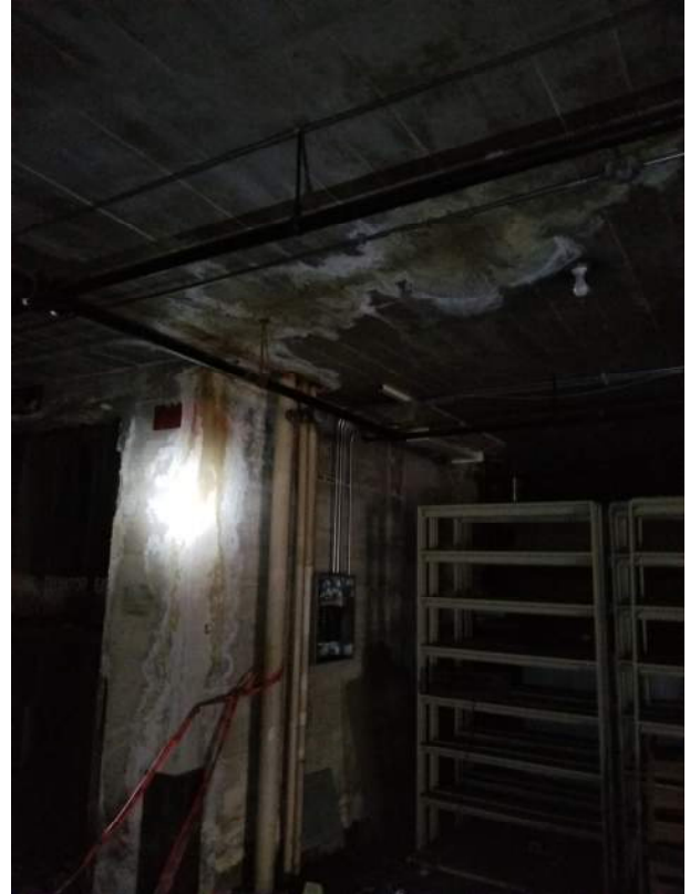
Corrosion of slab surrounding the freight elevator shaft
