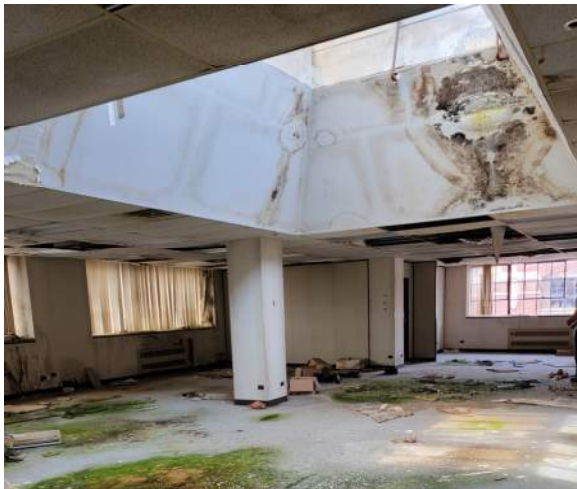
Mold and Corrosion @ Skylight
