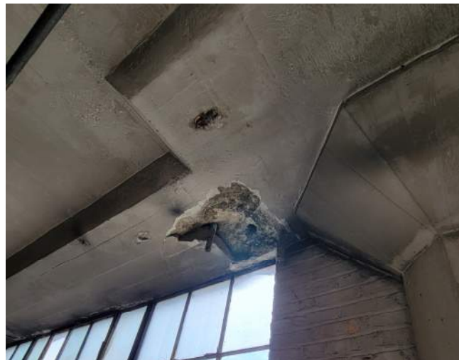
Spalling at North Spandrel Beam
