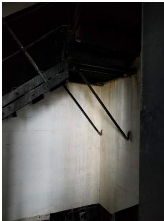
Rust from Metal Stair Structure
