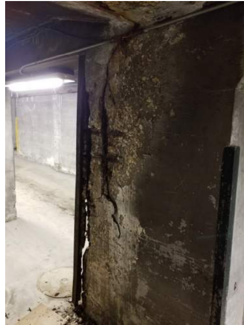
Deterioration of Link Column
