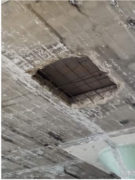
Cut Slab Near Column M.2
