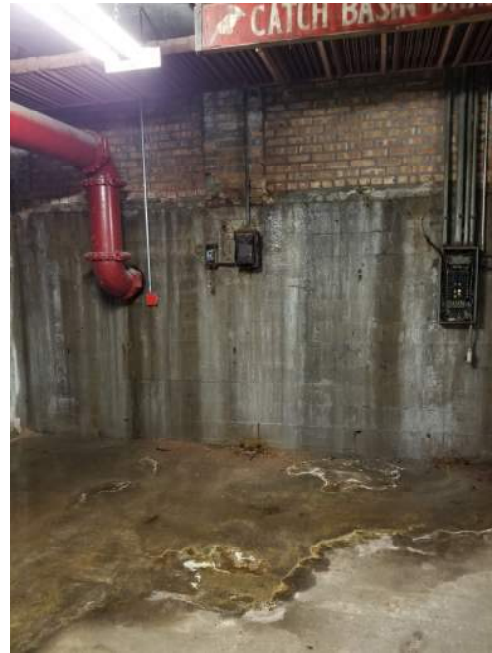
Water Leaks on Interior Face of Wall
