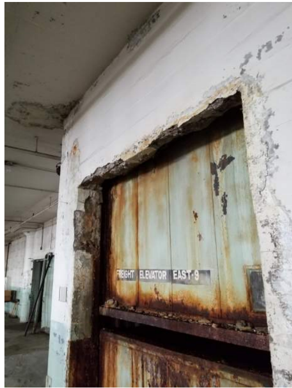
Deteriorated beam at freight elevator, and corrosion in adjacent 3 rd floor slab
