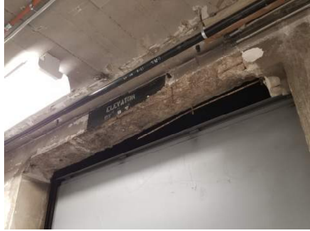
Cut Beam at Elevator B6
