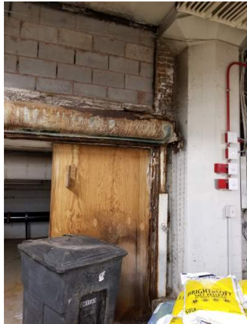
Deteriorated Masonry at Tunnel Entrance
