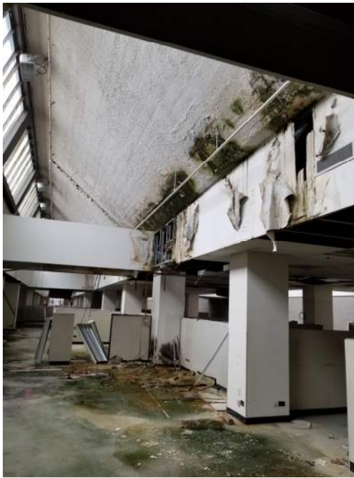
Water Damage at Skylights
