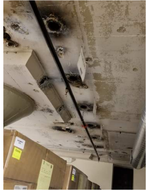
Plumbing Cores Through Concrete Slab
