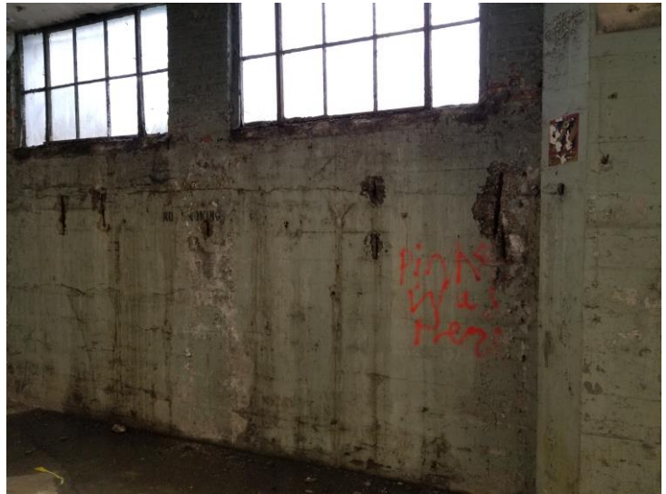
Exposed Rebar in Basement Wall
