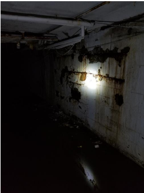
Deteriorated Rebar in West Building Tunnel
