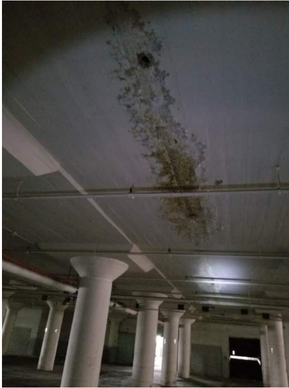
Corrosion visible on underside of 3 rd floor slab
