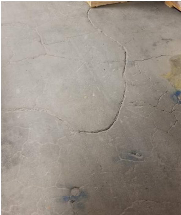
Floor Cracks at Level 5
