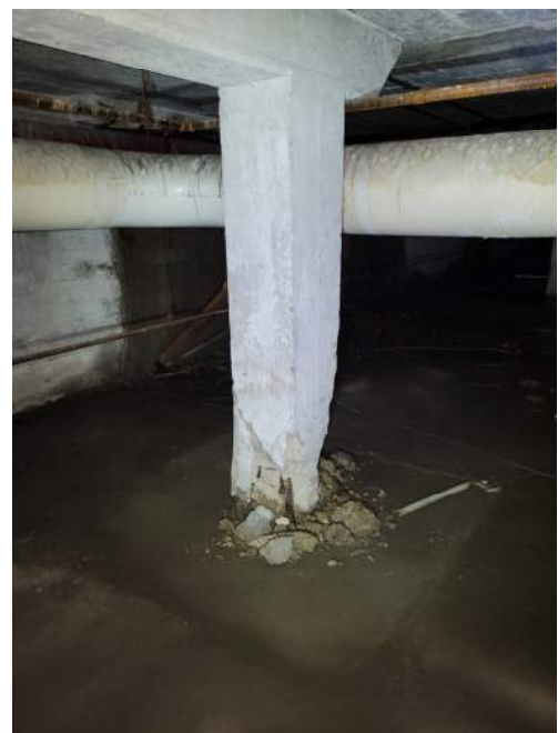
Concrete Post in Tunnel with Spalling at Base
