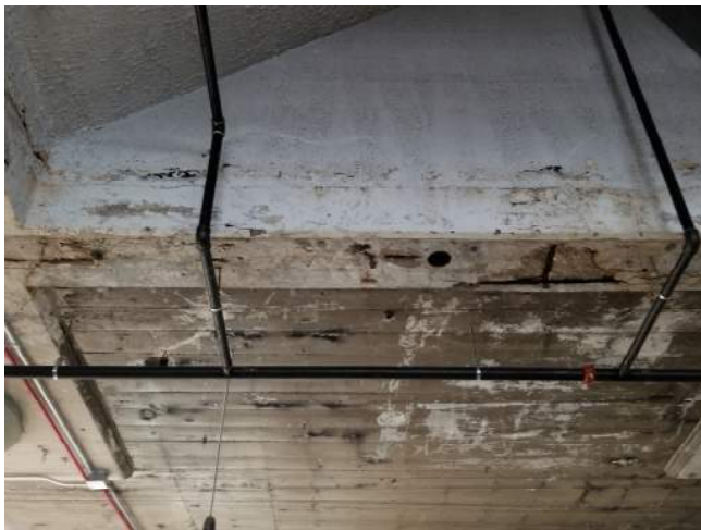
Exposed Rebar around Skylight
