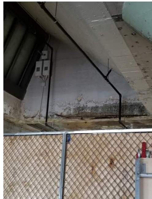
Exposed Rebar around Skylight
