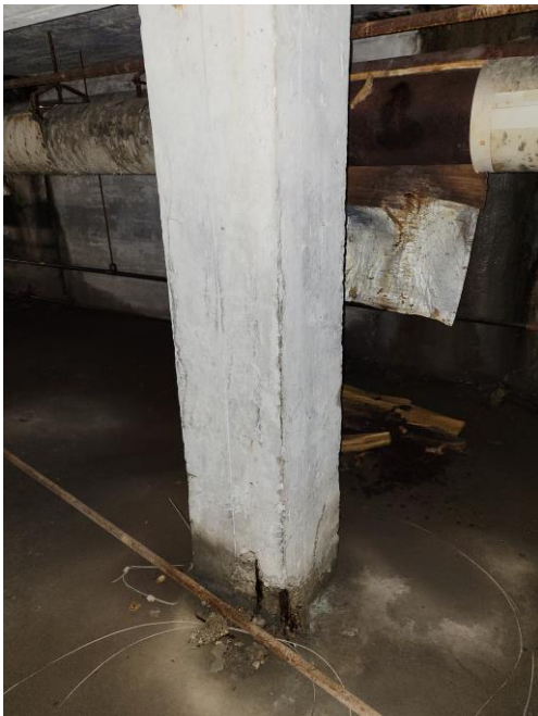
Concrete Post in Tunnel with Exposed Rebar
