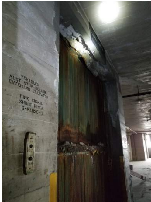
Elevator 13 Concrete Beam Deterioration
