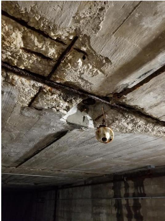
Exposed Rebar in Tunnel Slab
