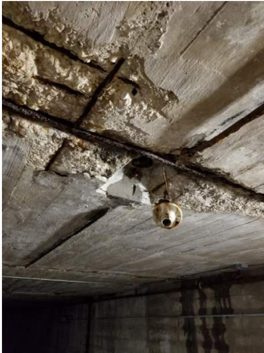
Exposed Rebar in Tunnel Slab
