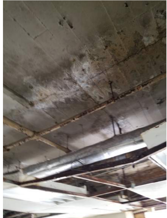
Corrosion visible on underside of Roof slab
