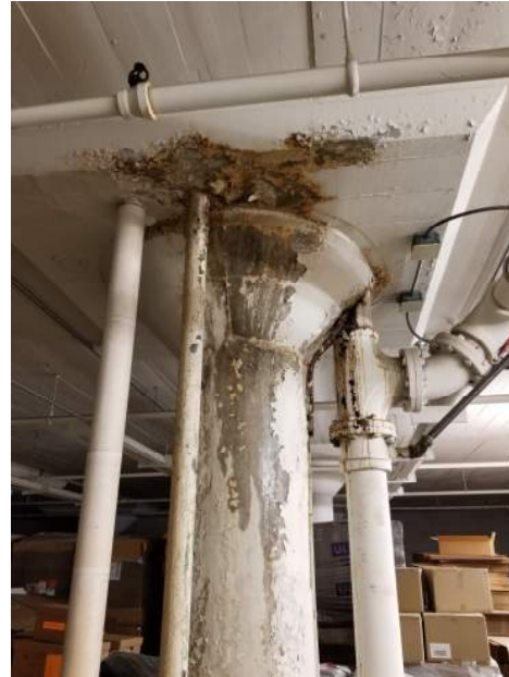
Water Damage at Column
