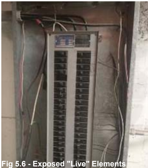
Fig 5.4 - Exposed "Live" Elements
