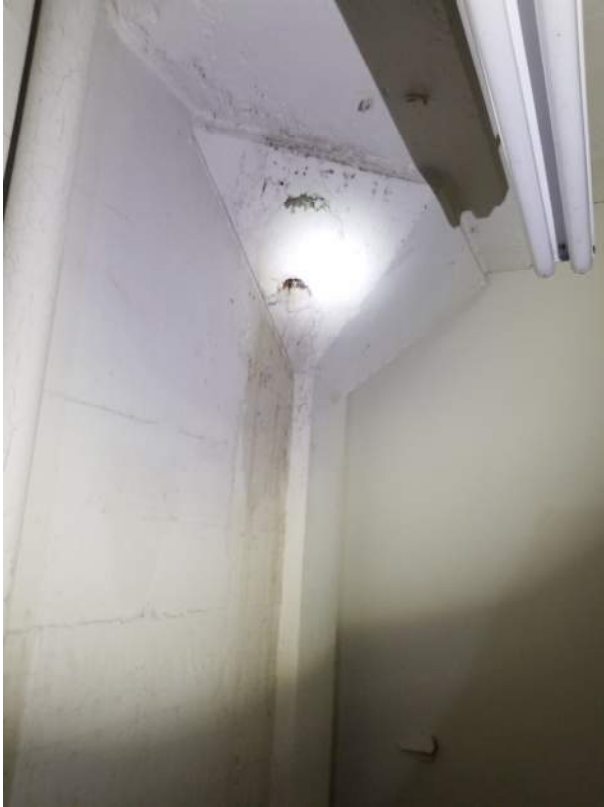
Active leak through column capital
