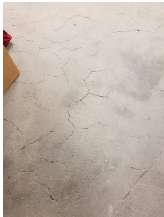
Floor Cracks at Level 5
