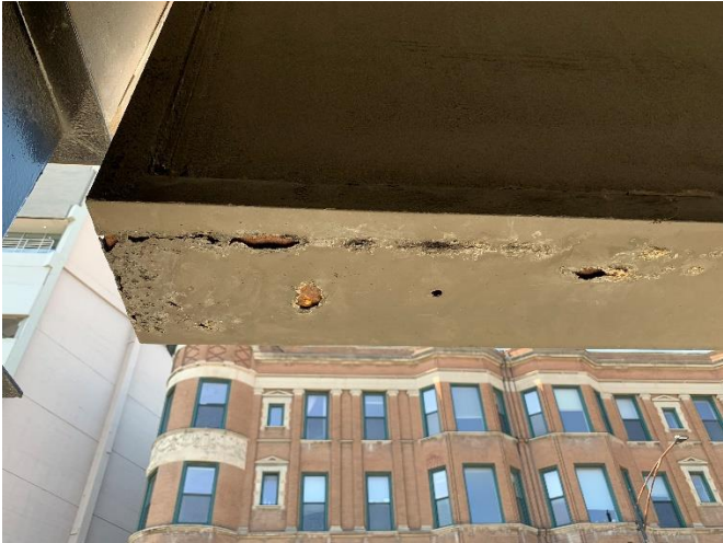
Pic 29 & 30: Sign enclosure shows corrosion.
