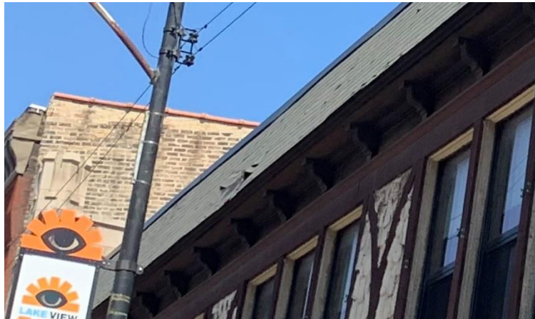
Pic 31: Shingle roof shows damage and deterioration and needs to be removed and replaced.
