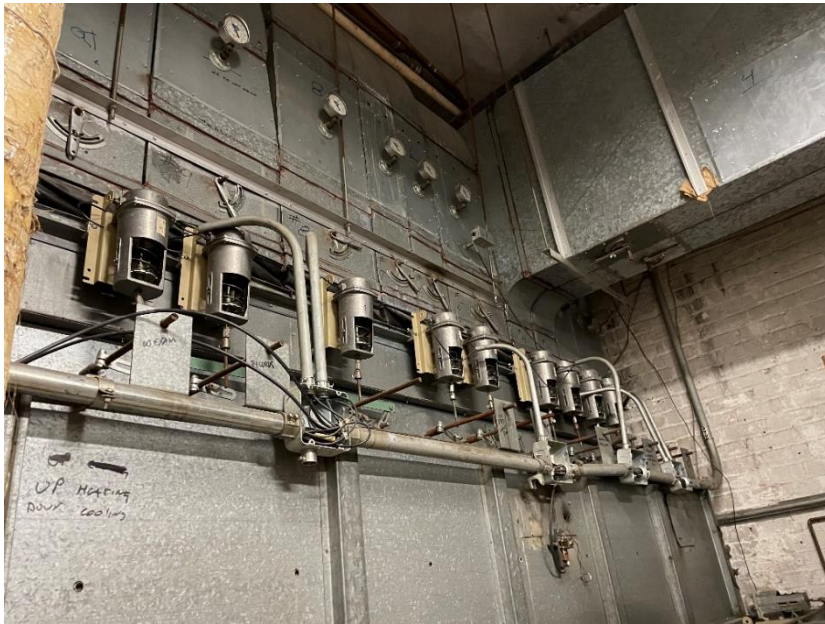
Existing AHU-1 Plenum with Damper Pneumatic actuator
