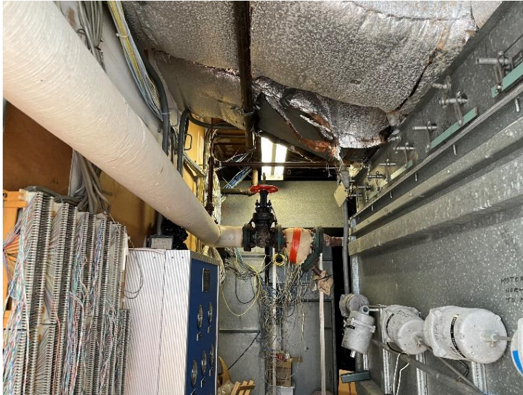
Existing AHU-2 Plenum Dampers Manually controlled Actuator are Disconnected
