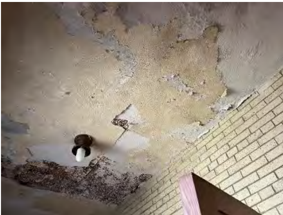
3.4.1.1.7 Ceiling in exit hall is damaged by moisture.
