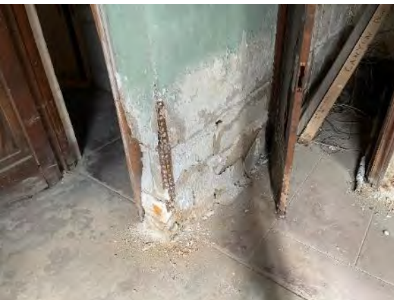
3.4.1.2.3 Basement wall is damaged by moisture
