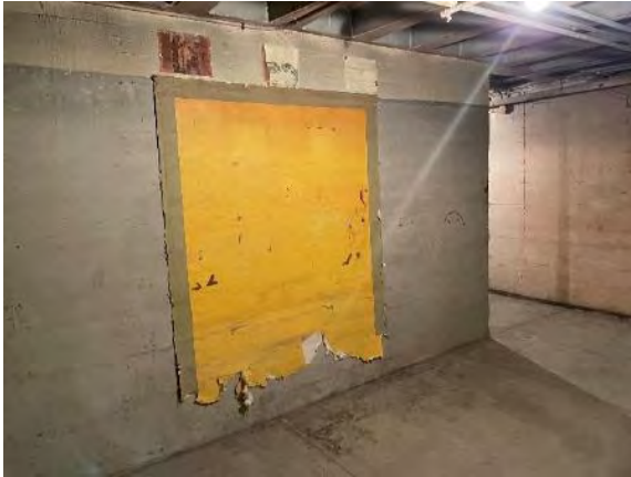
3.4.1.2.9 Dirt and debris built up in basement corridor. Some wall is damaged from moisture.
