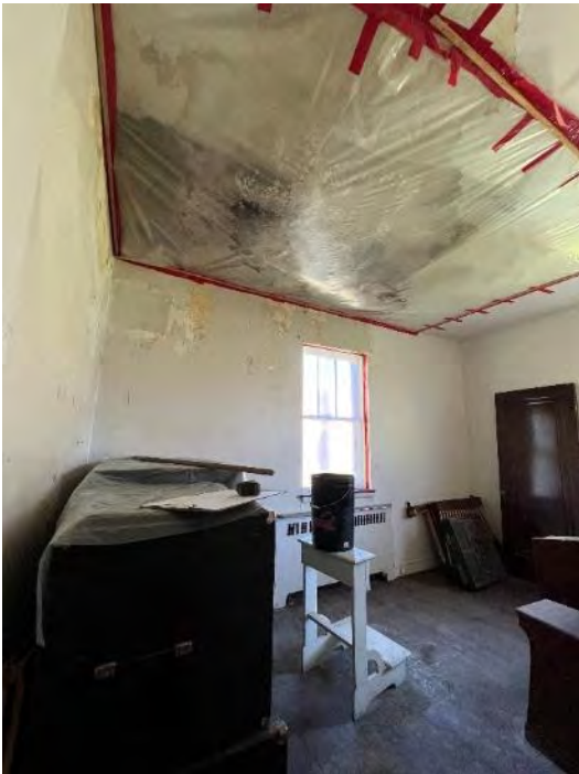
3.4.1.1.13 Room is damaged by water leaking through roof.
