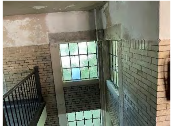
3.4.1.1.16 Window sills are damaged by moisture, and show some cracking.
