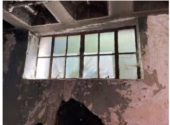
3.4.1.2.10 Windows in the basement are in poor condition.
