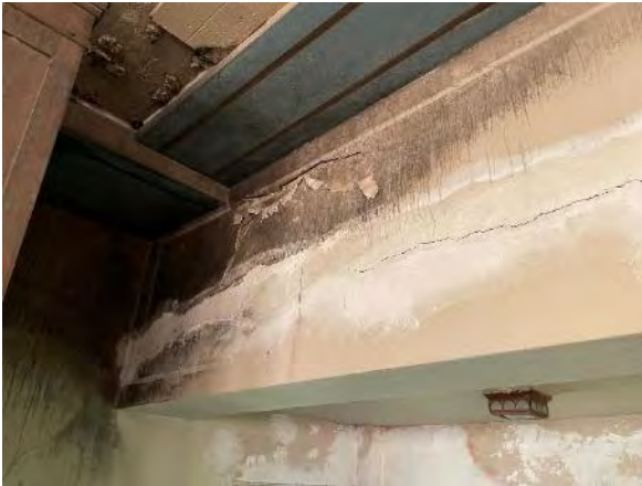
3.4.1.1.15 Concrete beam is damaged by moisture, potential mold growth.
