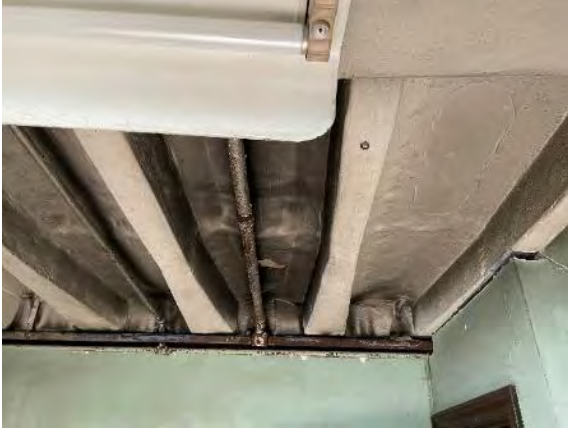
3.4.1.2.5 Basement ceiling and fire proofing is damaged
