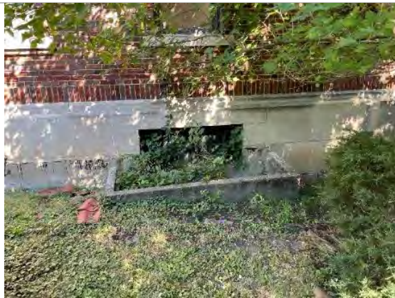
3.2.2.7 Light well is covered with dirt and plants.
