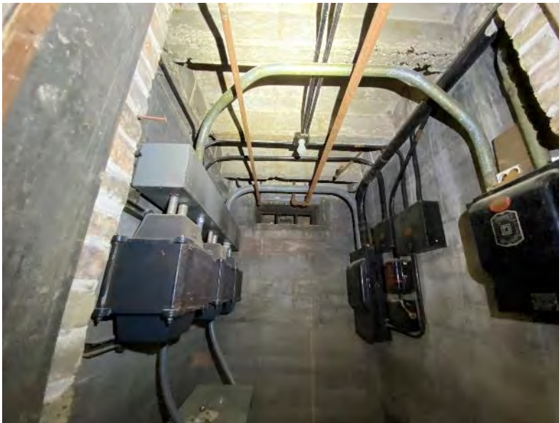
3.3.4.4.2.3 Electrical Room with insufficient clearances and out of date/non-function equipment.
