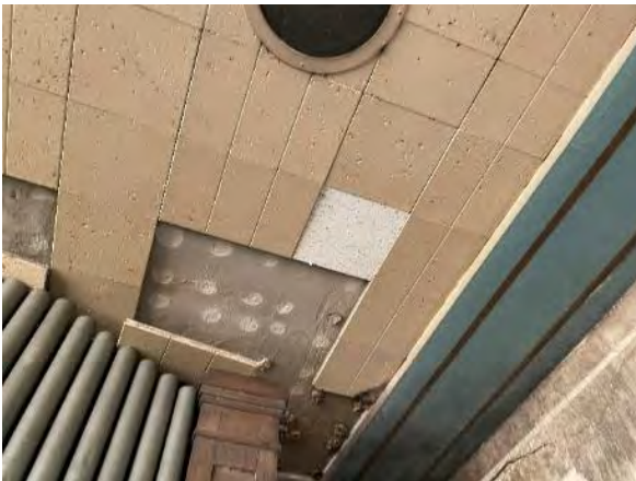
3.4.1.1.17 Ceiling tiles are missing in the choir area.
