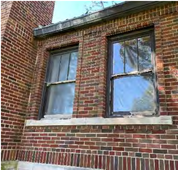
3.2.3.1 Existing Double Hung windows in poor condition
