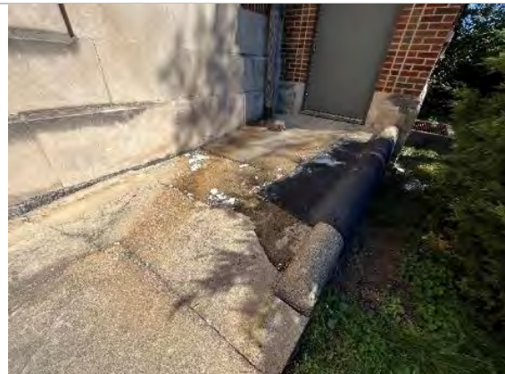
3.2.2.8 Concrete paths into exit doors are damaged.
