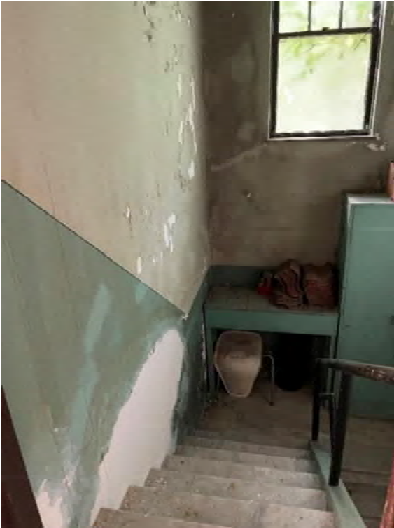
3.4.1.2.1 Stairs down to basement are in good condition; however, it is not ADA compliant
