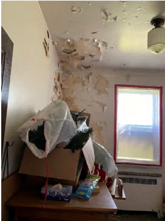
3.4.1.1.11 Ceiling and dry wall in bedroom shows damaged by moisture.
