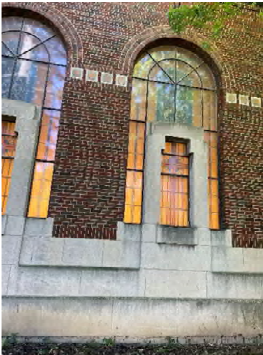
3.2.3.3 Existing stained-glass windows with limestone inlay elements
