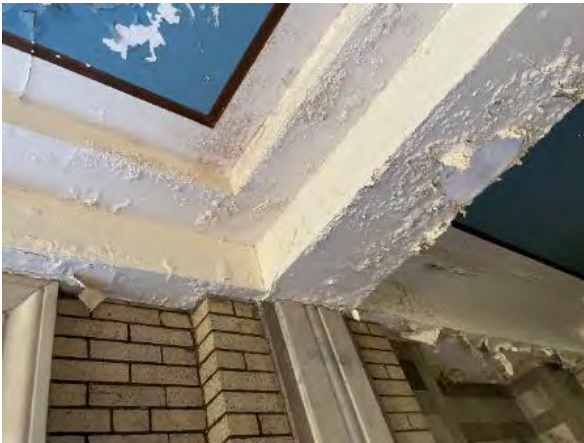
3.4.1.1.3 Plaster ceiling in the vestibule is not in good condition.
