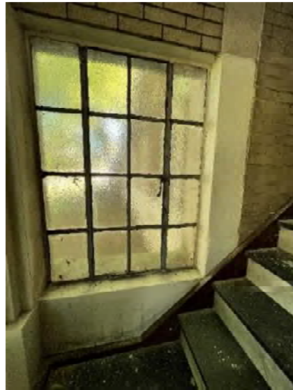
3.2.3.2 Existing divided light casement windows in poor condition
