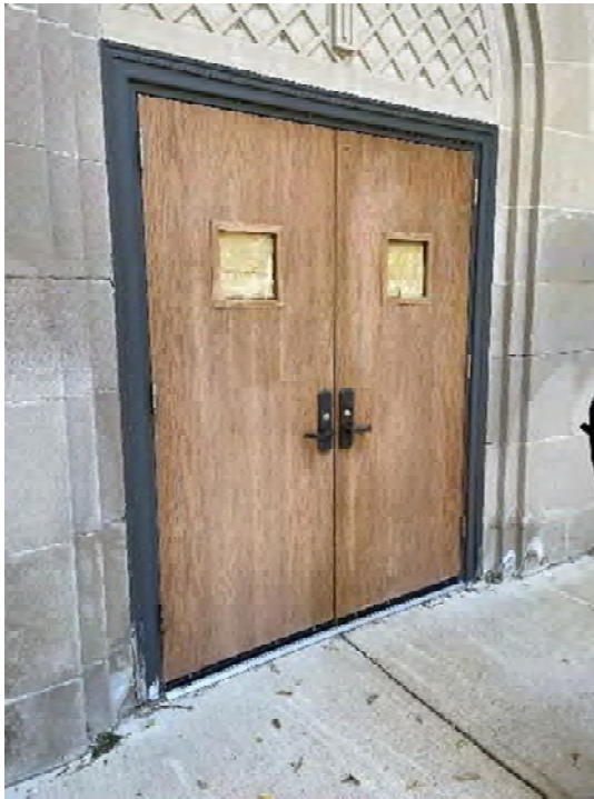
3.2.4.1 Main Entry Door, Hardware in fair condition but glazing is damaged.
