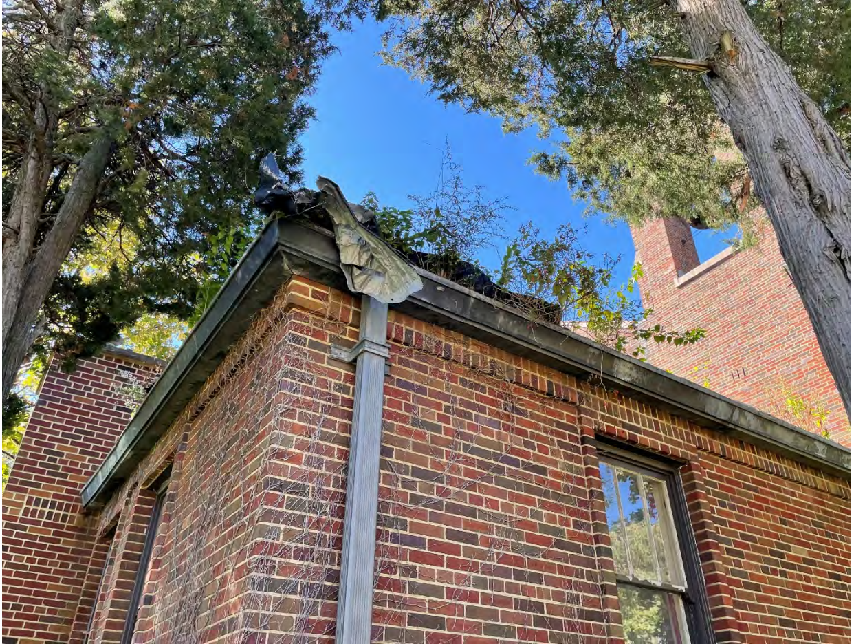
3.2.7.3 Overgrowth and damaged sheet metal on north west corner of the building
