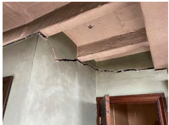
3.4.1.2.4 Wall is cracking.
