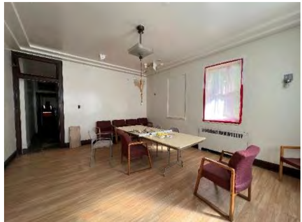
3.4.1.1.8 Office floor is in good condition. Ceiling shows damaged by moisture in the corner.
