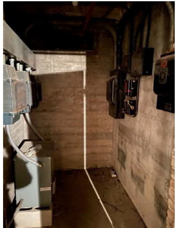
3.4.1.2.8 Dirt and debris built up in basement. Wall showed damaged from moisture.
