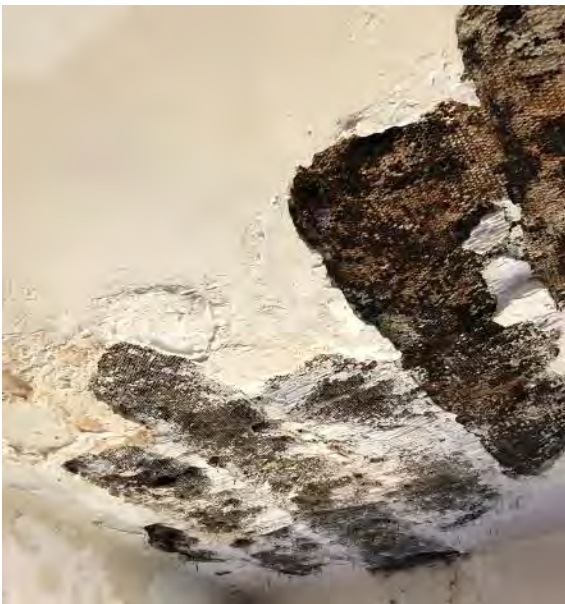
3.2.1.3. Ceilings show signs of significant water damage. This is an indication that water damage to the roof structure is expected. It is expected that the roof be composed of timber. Structural framing system should be inspected (or replaced) to ensure no structural deficiencies, which will require selective demo.
