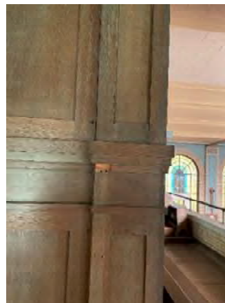
3.4.1.1.18 Some piece of trim on millworks is missing.
