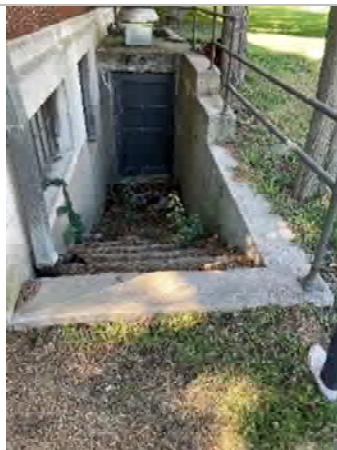
3.2.2.9 Dirt and debris built up along the wall, steps and door of basement exit door.
