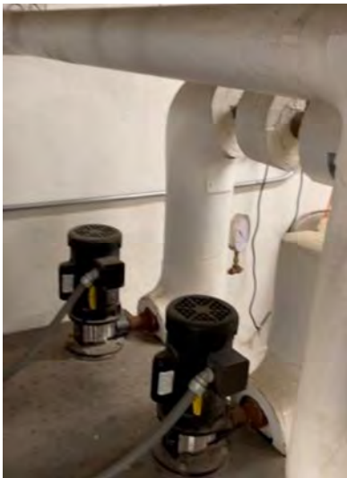
3.3.2.2. Existing condensate return station in basement.
