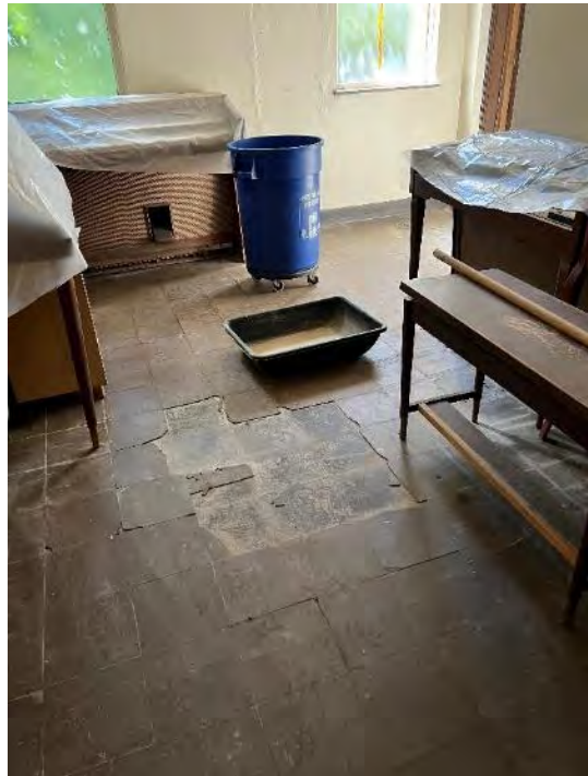
3.4.1.1.14 Floor tiles are missing.
