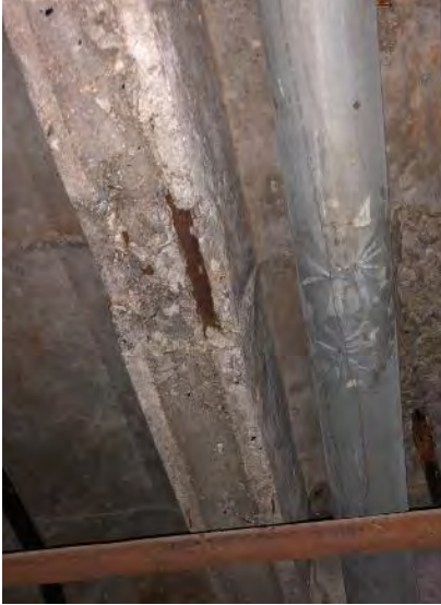
3.2.1.2. First floor framing above basement is composed of concrete slab on concrete beams
