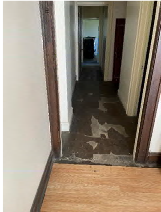
3.4.1.1.12 Floor tiles are missing in the hall way from office to bedrooms.
