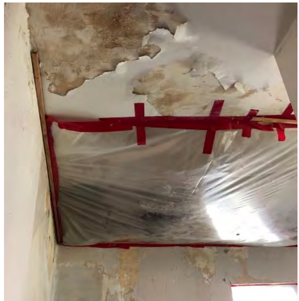
3.2.1.3. Ceilings show signs of significant water damage. This is an indication that water damage to the roof structure is expected. It is expected that the roof be composed of timber. Structural framing system should be inspected (or replaced) to ensure no structural deficiencies, which will require selective demo.
