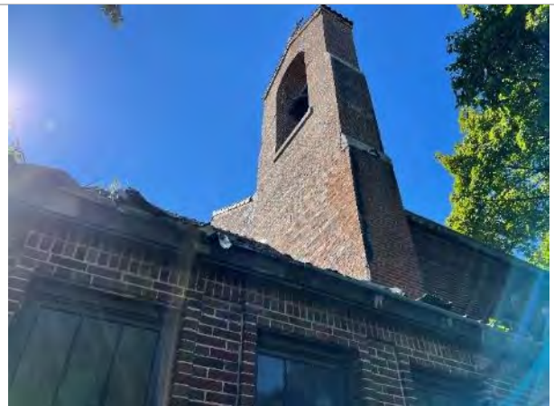
3.2.2.10 Cracking on bell tower allows water to leak through brick.
