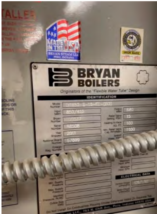
3.3.2.1 Nameplate of existing steam boiler in basement.
