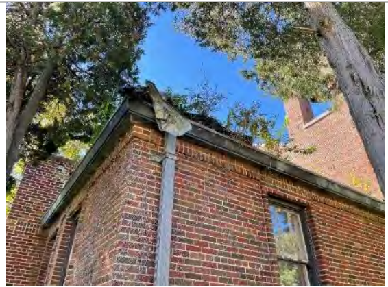
3.2.2.6 Plants and dirt built up on the gutter of the building.
