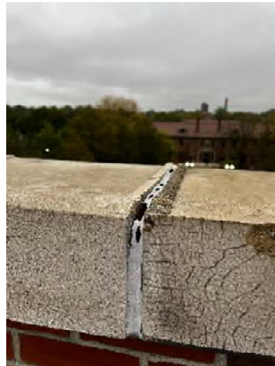
3.2.7.8 Sealant at Limestone coping
