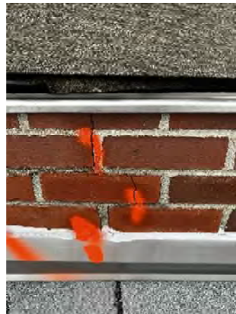
3.2.7.4 Masonry cracking at Masonry Parapet
