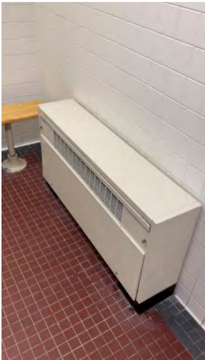
3.3.2.3 Existing terminal cabinet unit heater
