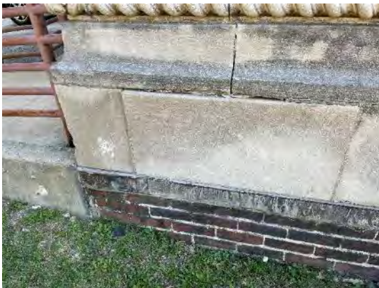
3.2.3.6 Rust/Moisture damage visible at masonry base wall
