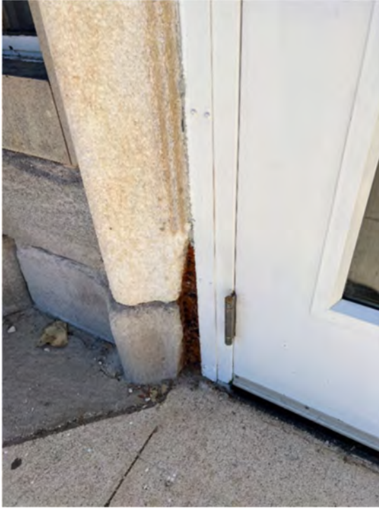
3.2.3.8 Lime stone base got rusted by moisture/ water
