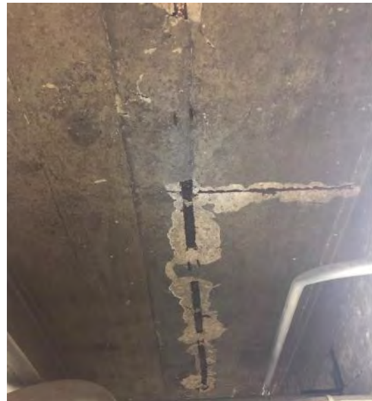
3.2.2.2 Concrete beam with large crack
