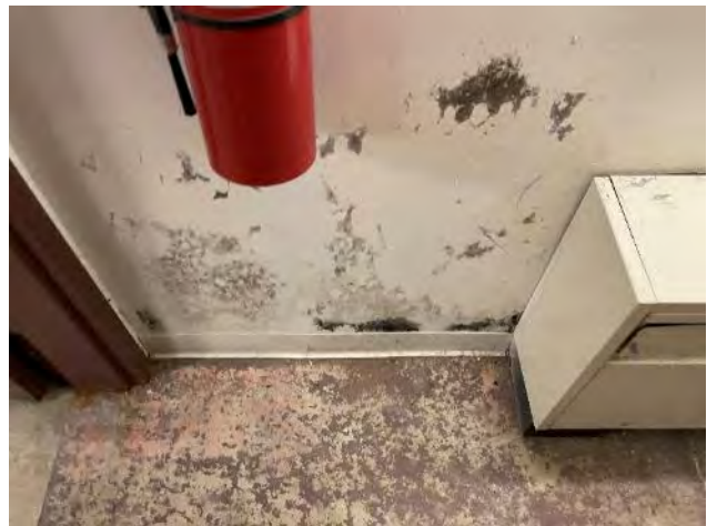
3.4.1.1.1 Dry wall is missing from water damage in the basement. Basement is damp from water penetration.
