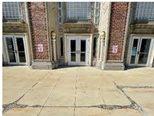
3.1.4.2 Eastern, concrete entrance plaza is deteriorated. Associated curb ramp is non-conforming in the vehicular drop-off area
