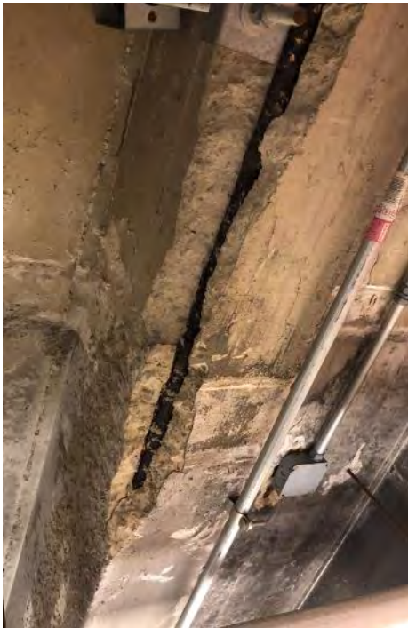
3.2.2.1. Concrete beam with spalling
