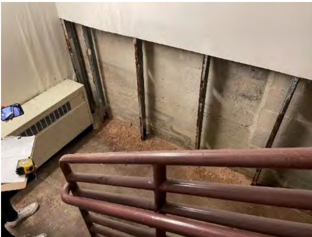
3.4.1.1.1 Dry wall is missing from water damage in the basement. Basement is damp from water penetration.
