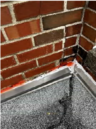
3.2.7.7 Damage to sealant and flashing
