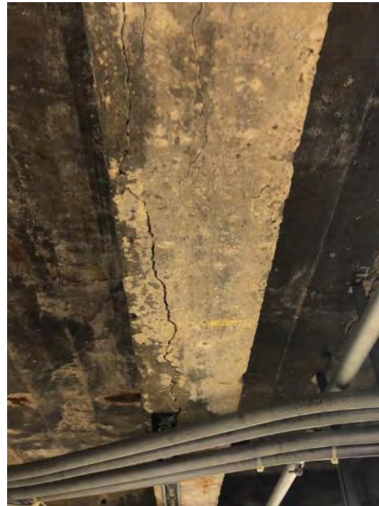
3.2.2.2 Concrete beam with large crack
