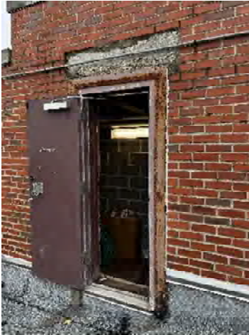
3.2.7.5 Access Door at Roof, door and frame in poor condition
