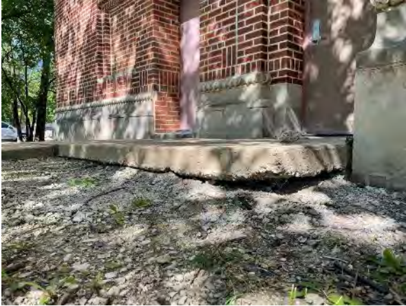
3.1.4.3 Settlement of earth and washout are compromising the sidewalk at the southern entrance.
