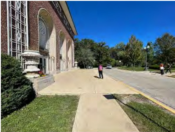
3.1.4.1 The southeastern landscape area has settled, exposing the side of the sidewalk
