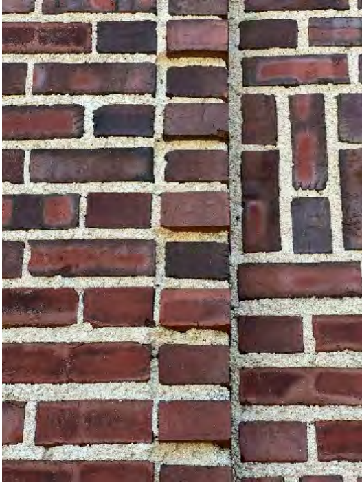
3.2.3.4 Brick shows aging and cracking. Brick's joints are wearing out because of weather condition on site.
