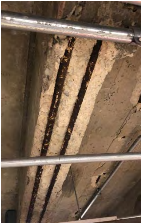
3.2.2.1. Concrete beam with spalling
