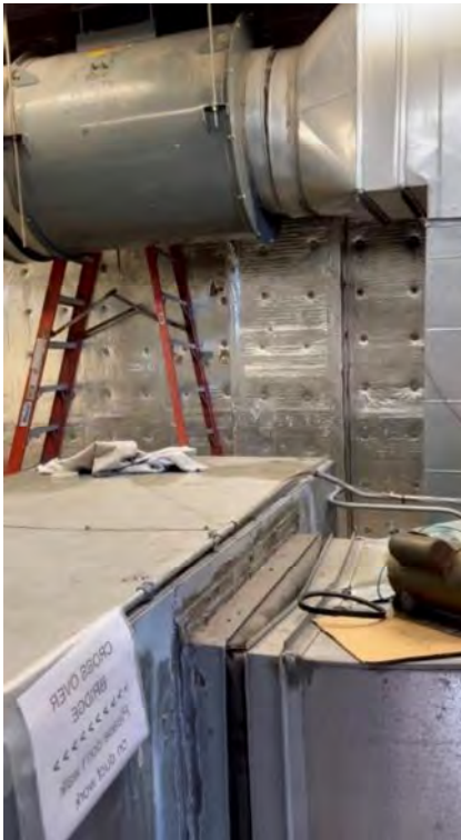
3.3.3.1 Existing penthouse air handler and return fan
