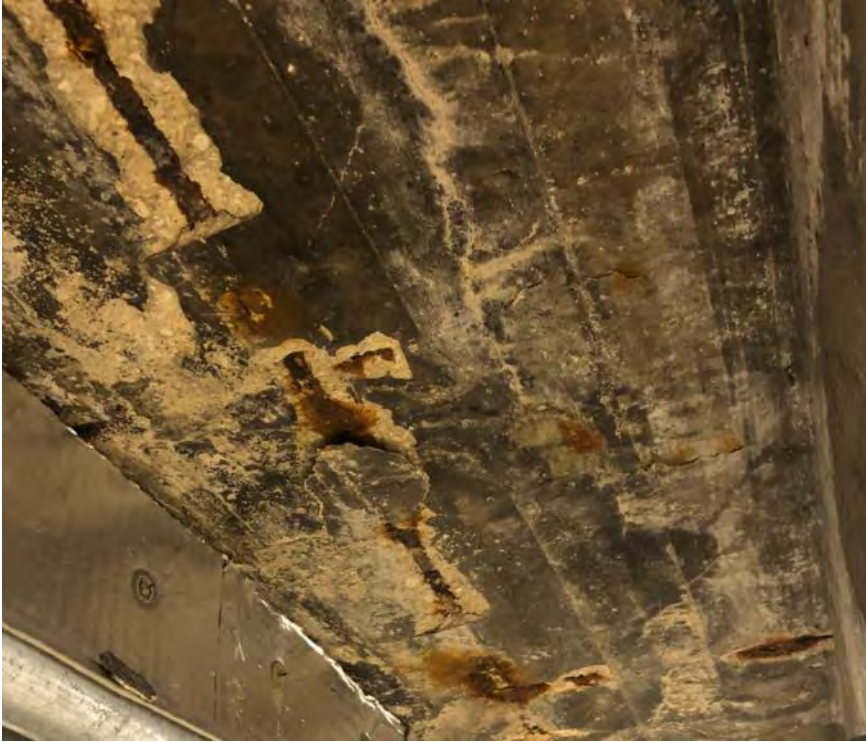
3.2.2.5. Concrete slab with concrete spalling
