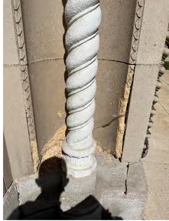
3.2.3.9 Lime stone décor feature got damage by moisture/ water
