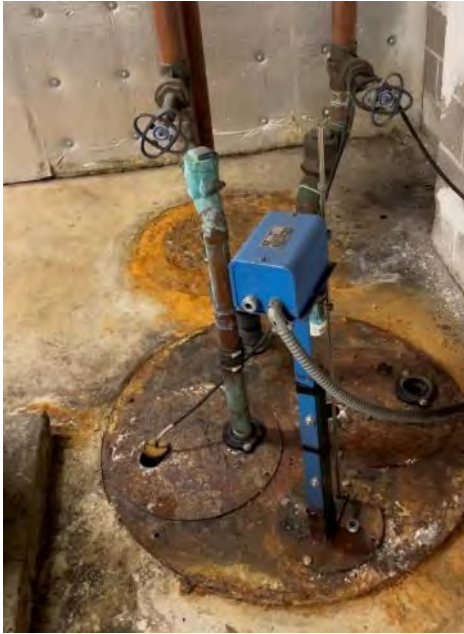
3.3.1.3 Existing basement sewage ejector
