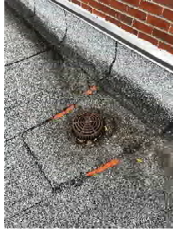
3.2.7.6 Damage to roof membrane at Roof Drain
