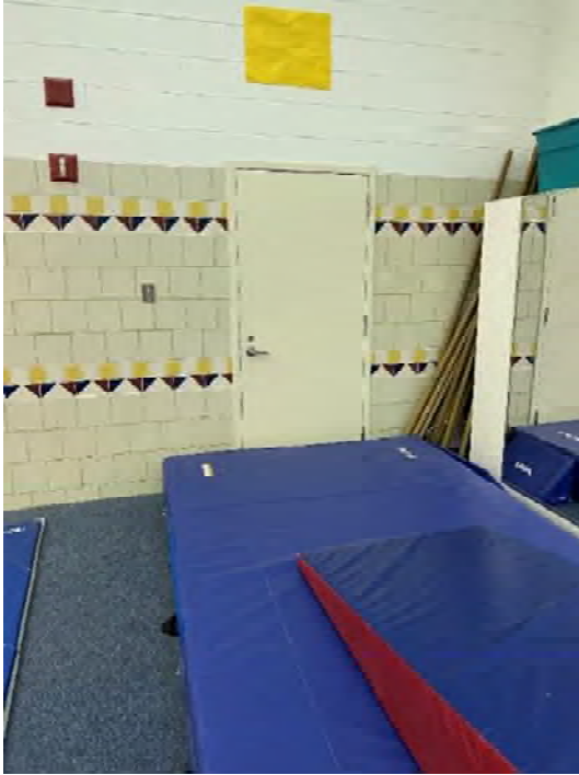
3.4.1.1.6 Level 1 and Level 2 Doors appear to typically painted hollow metal with ADA compliant hardware
