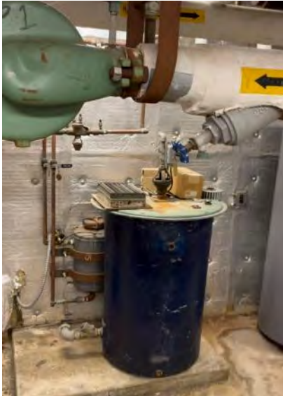
3.3.2.2 Existing basement heating pump and glycol fill station.
