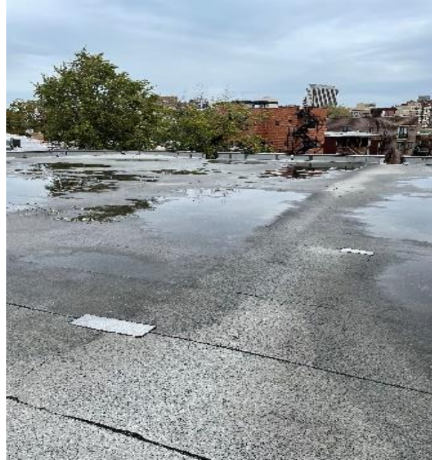
Compromised thermal and moisture protection
