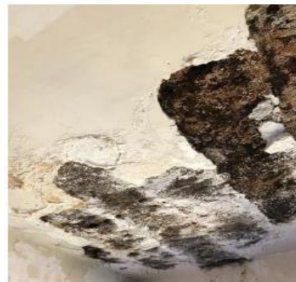
3.2.1.3. Ceilings show signs of significant water damage. This is an indication that water damage to the roof structure is expected. It is expected that the roof be composed of timber. Structural framing system should be inspected (or replaced) to ensure no structural deficiencies, which will require selective demo.
