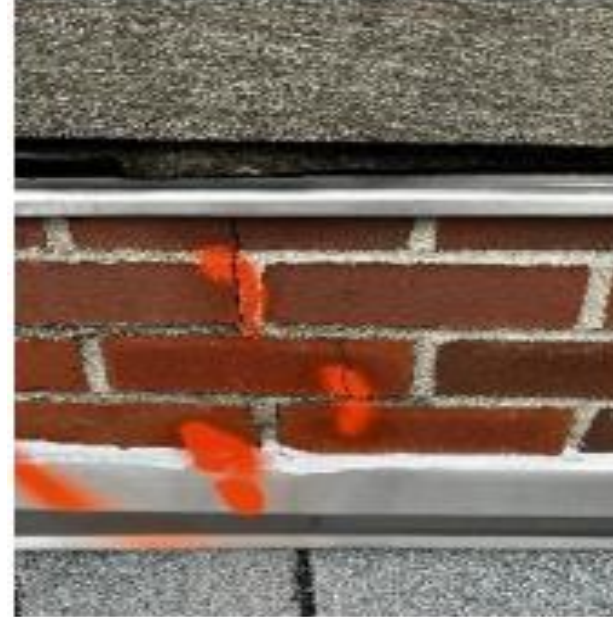
3.2.7.4 Masonry cracking at Masonry Parapet
