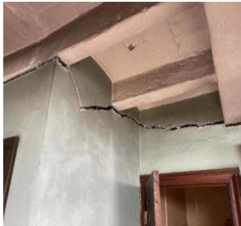
3.4.1.2.4 Wall is cracking.
