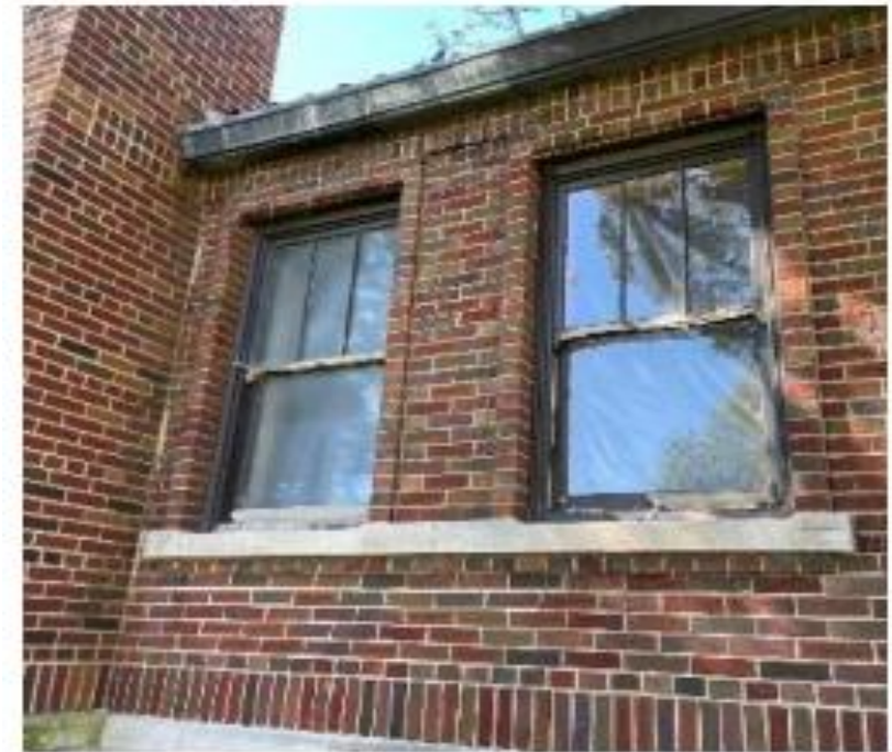
3.2.3.1 Existing Double Hung windows in poor condition
