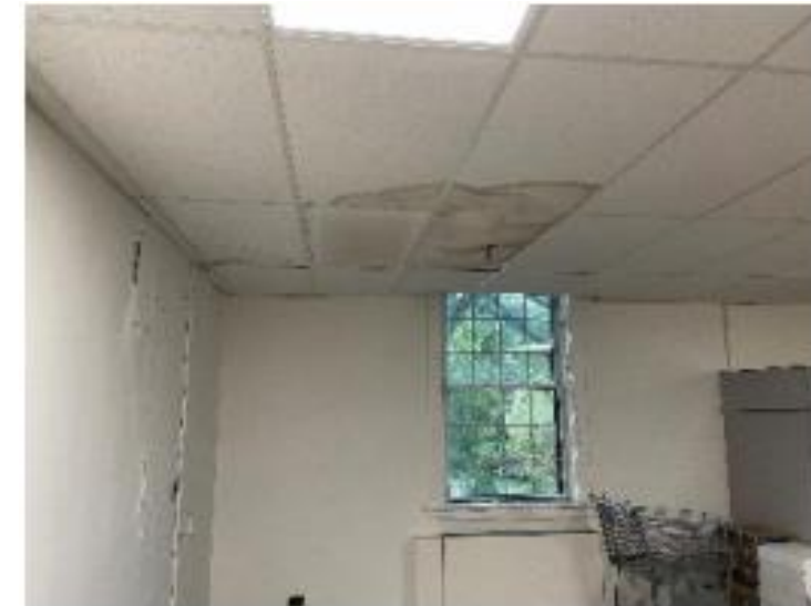
3.4.2.32 Moisture damage at ceiling in Room 210. Active leaking is ongoing at Room 210.
