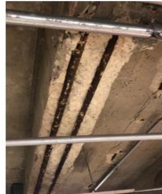
3.2.2.1. Concrete beam with spalling
