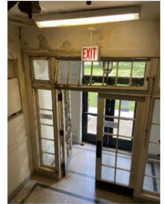
3.4.1.1.2 Door Hardware at the majority of Office Doors is not Accessible.
