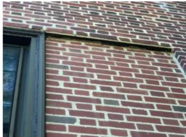
3.2.1.5 Steel lintels spanning over 1 st and 2 nd floor windows on east and west ends of building show signs of rust and corrosion.
