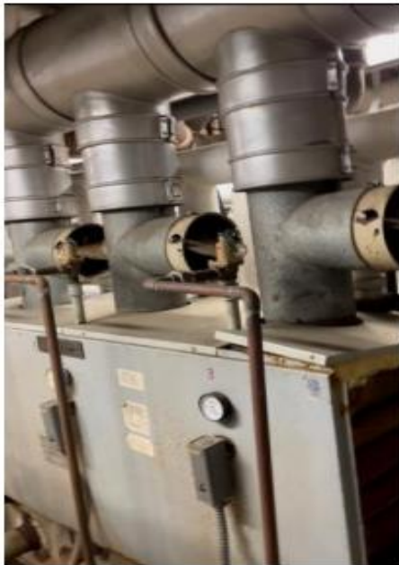
3.3.2.1 Existing basement boiler
