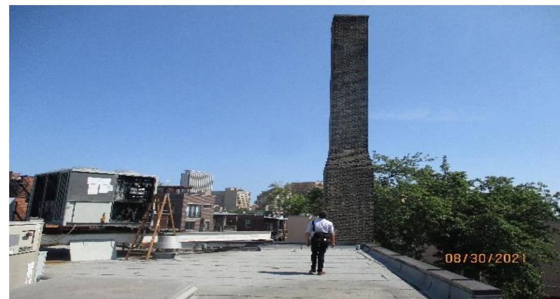
Deteriorating masonry chimney and existing mechanical equipment
