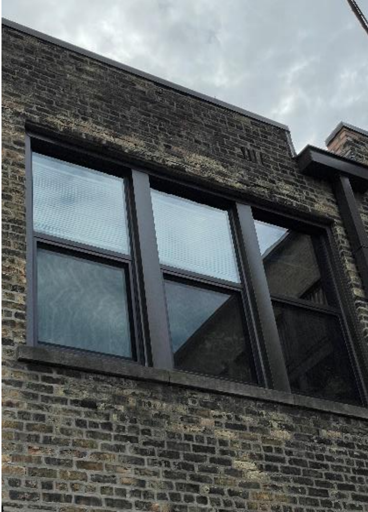
Deteriorating Lintels
