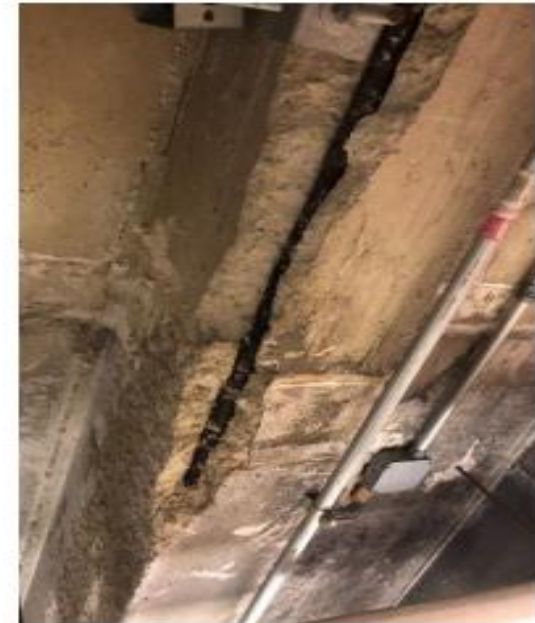
3.2.2.1. Concrete beam with spalling
