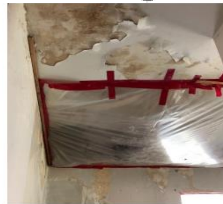
3.2.1.3. Ceilings show signs of significant water damage. This is an indication that water damage to the roof structure is expected. It is expected that the roof be composed of timber. Structural framing system should be inspected (or replaced) to ensure no structural deficiencies, which will require selective demo.
