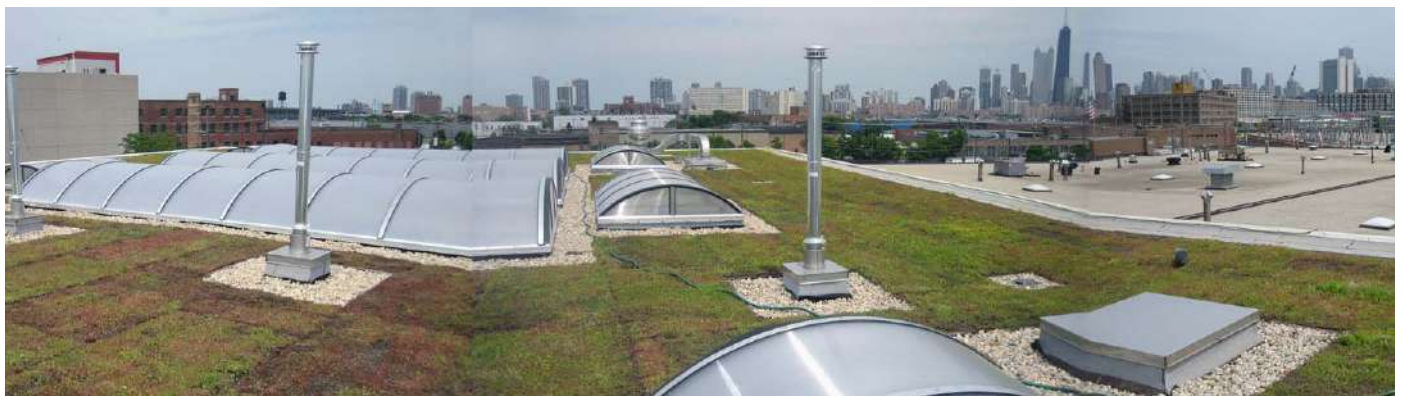
Vegetative Roof and Refurbished Skylights at Training Center
