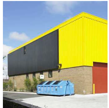
Solar Wall on South Facade
