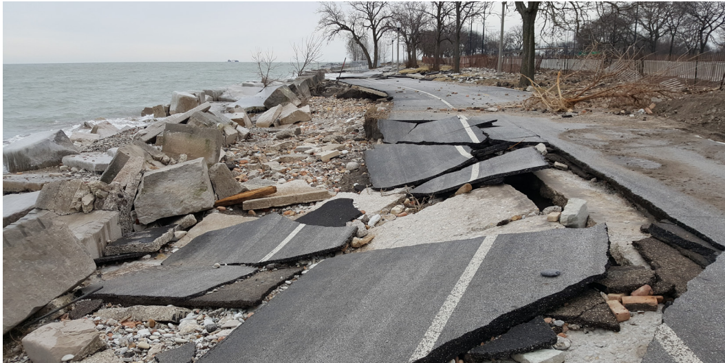
Destroyed lakefront path due to wave action
