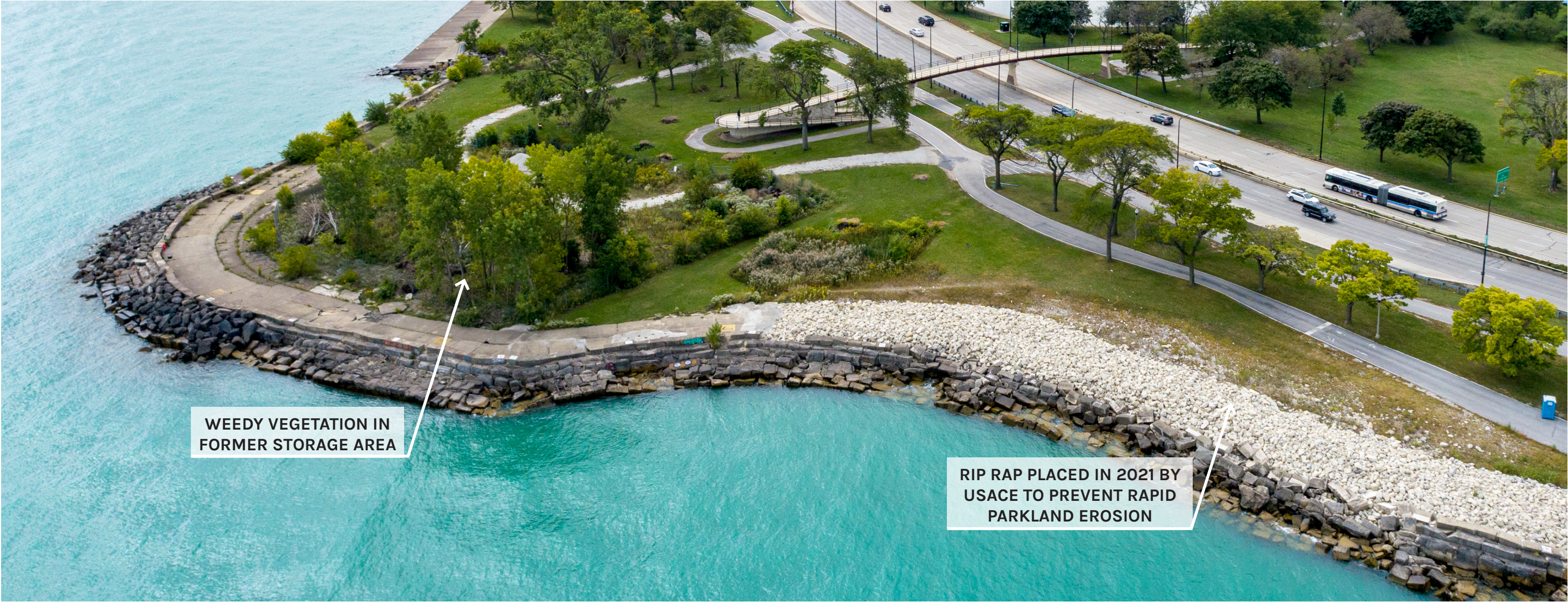
Deteriorated landscape at the landing of the existing 51st Street pedestrian bridge and rip rap for temporary erosion protection.
