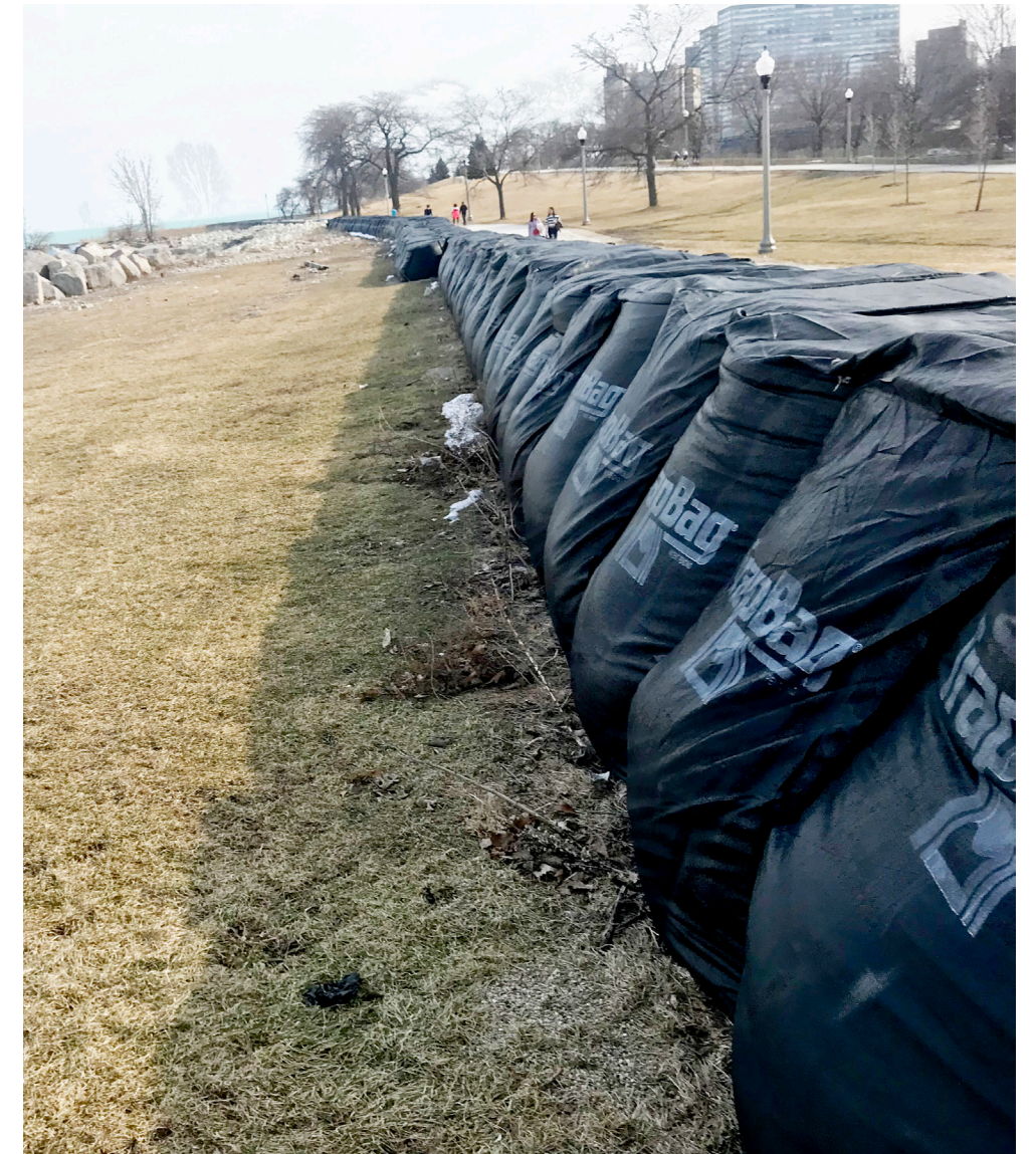
TrapBags installed as temporary flood protection
