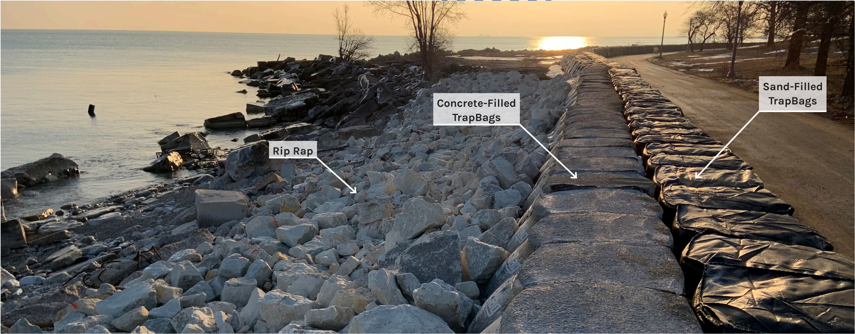
Deteriorating shoreline separated from pedestrian trail with temporary measures of rip rap and TrapBags.
