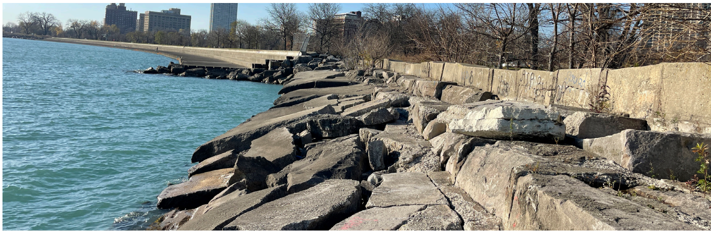
51st St existing concrete installed in 1970 is deteriorated and limits safe pedestrian access to water
