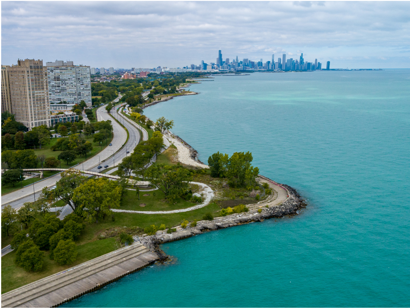
Aerial of Morgan Shoal project area
