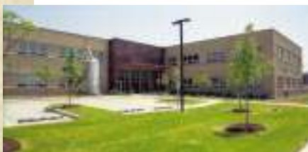
Photos: (left) Southwest Mental Health Center; (middle) Solar panels on roof of Chicago Center for Green Technology; (bottom) Chicago Center for Green Technology
