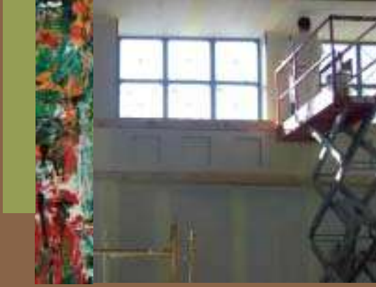
Painting the interior of future West Englewood Branch Library
