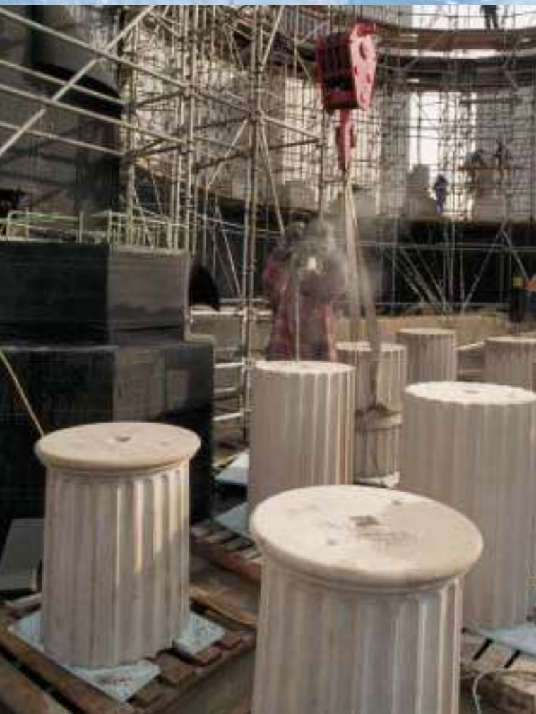
Millennium Park Peristyle under construction
