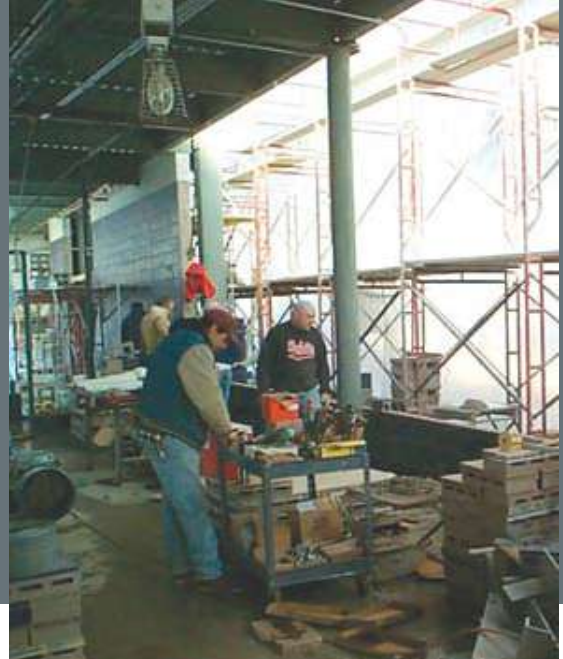
Construction at Hayes Park Natatorium
