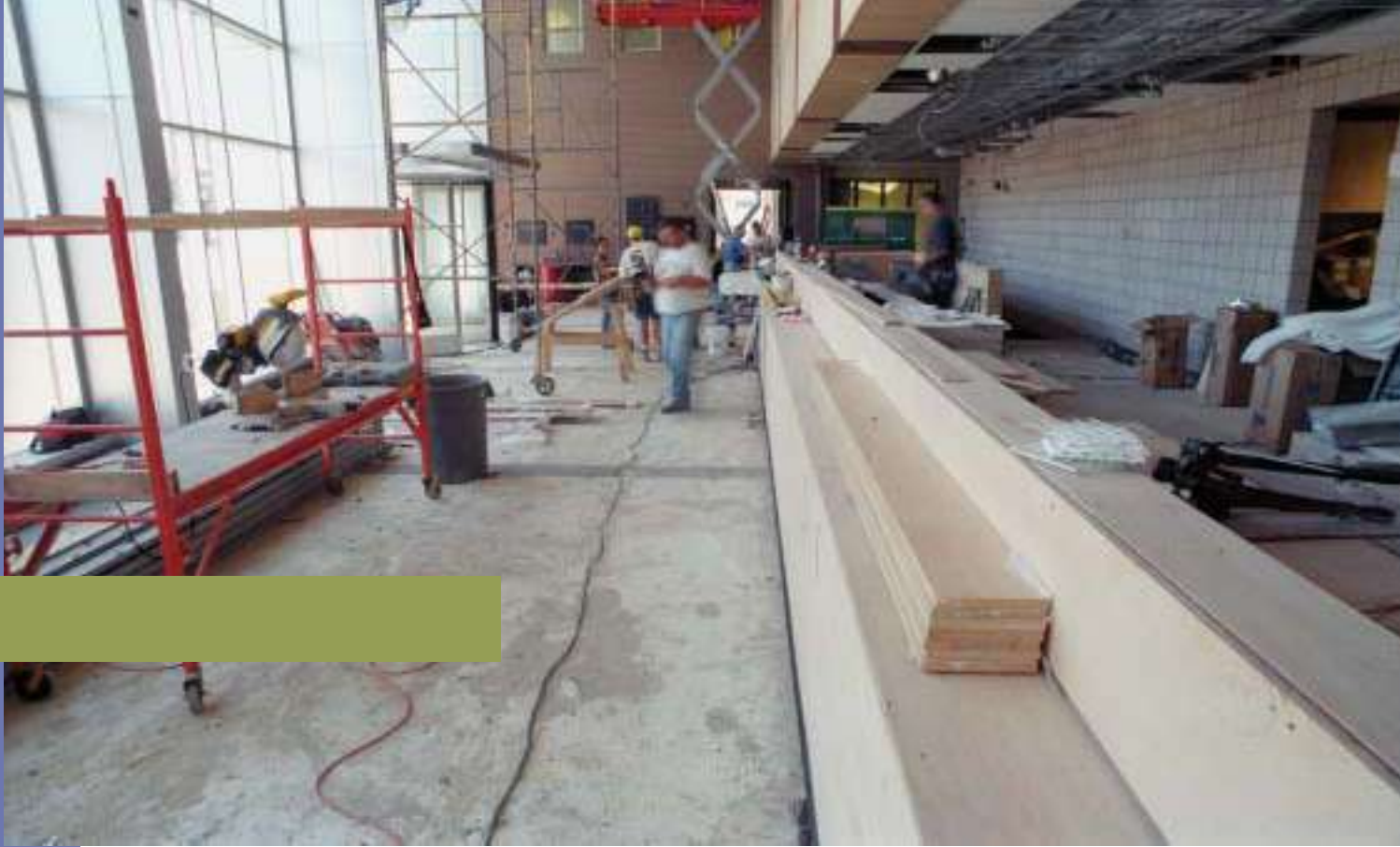
Interior construction at 20th District
