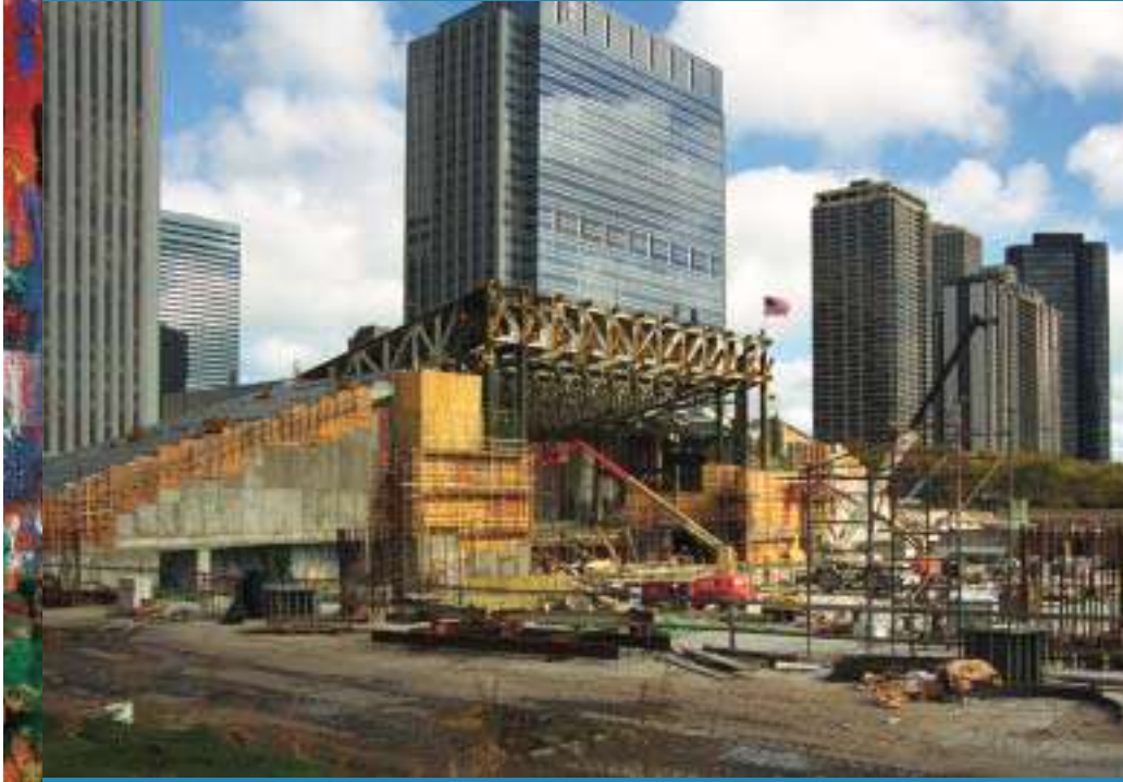
Gebry band shell under construction
