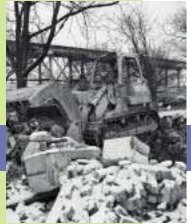
Demolition at future site of new Kennedy-King College Campus
