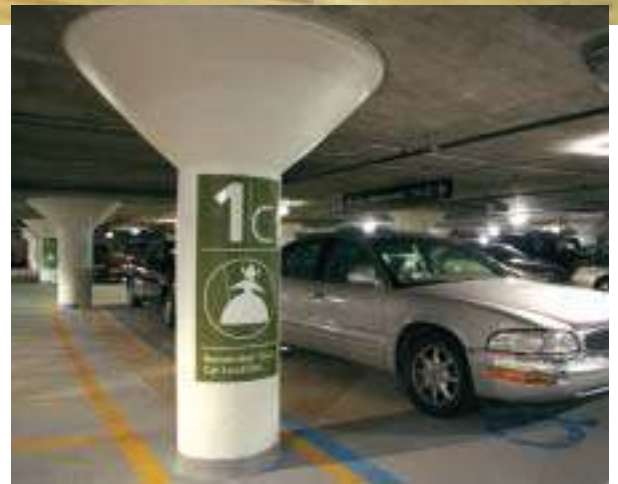
Grant Park South underground parking
